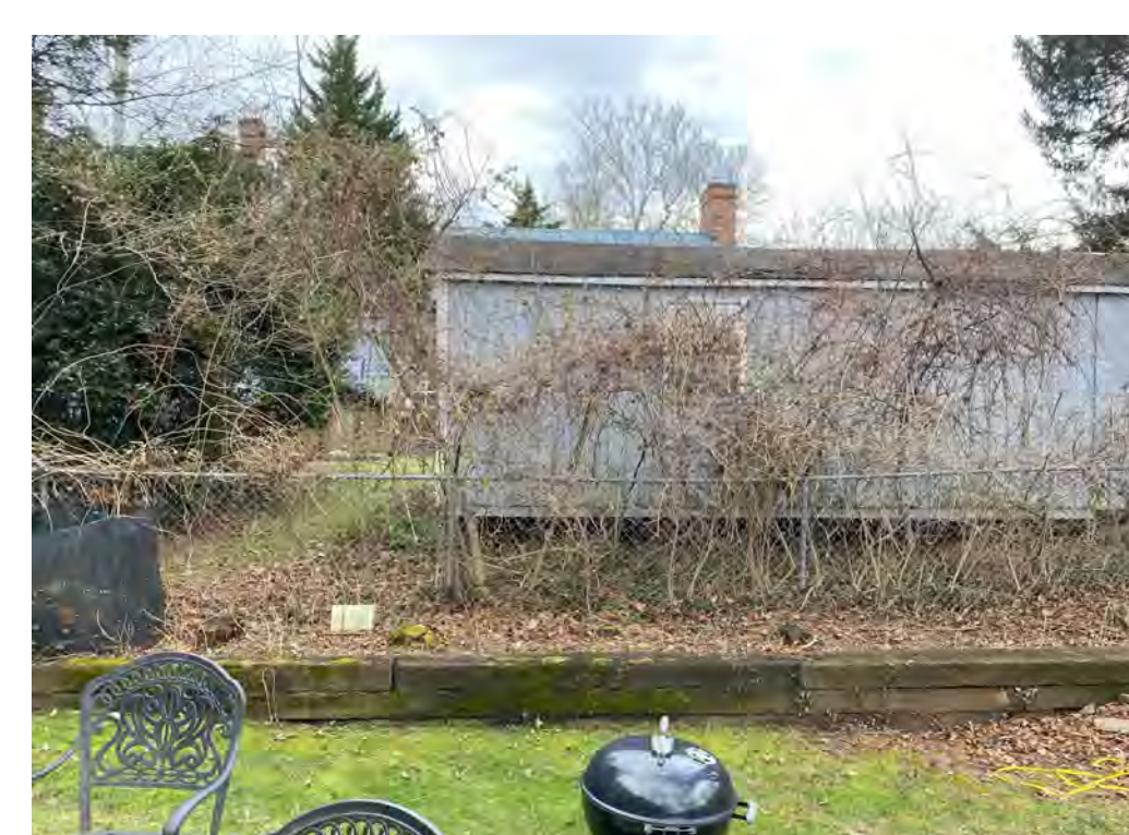
Partial view of Existing Timber Retaining Wall to be Replaced w/ 6x6 P.T. Timbers
