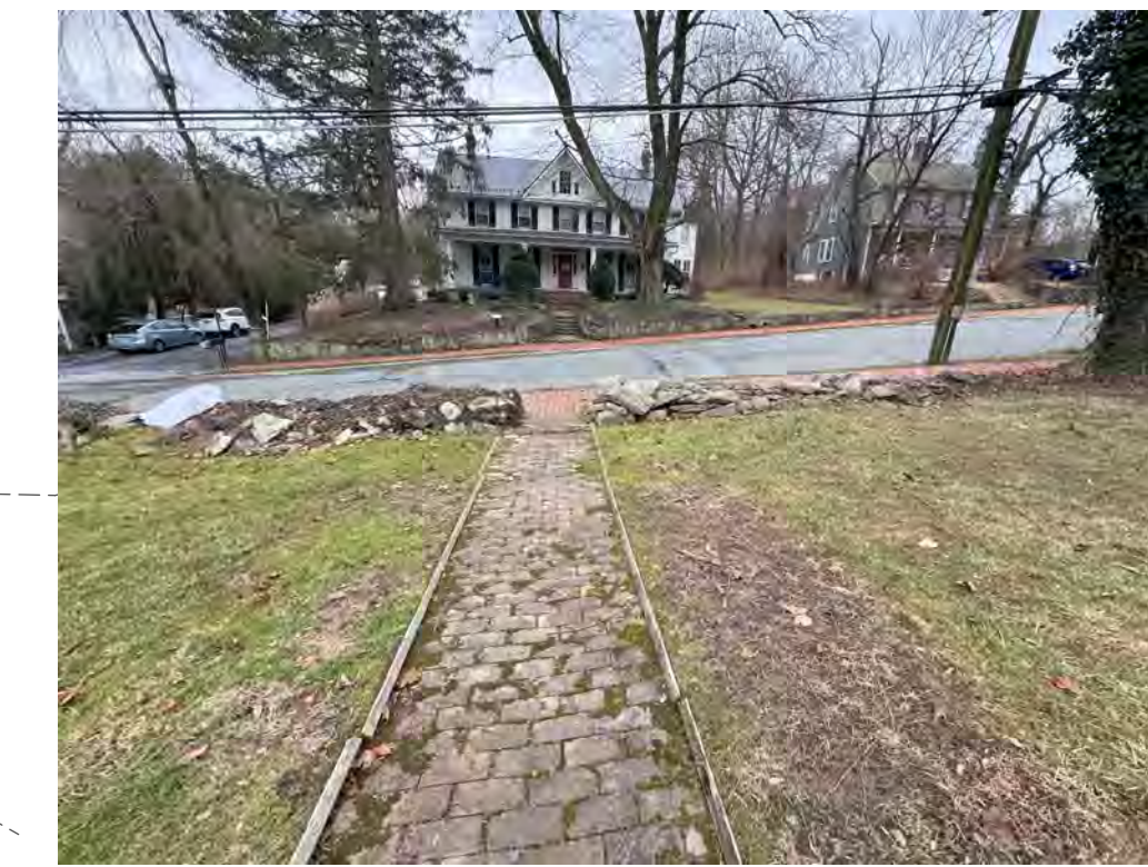
View of Brick Front Walk and Existing Stone Wall. Wood Edging along Brick to be Removed. Brick walk to be Slightly Raised + Reset.
