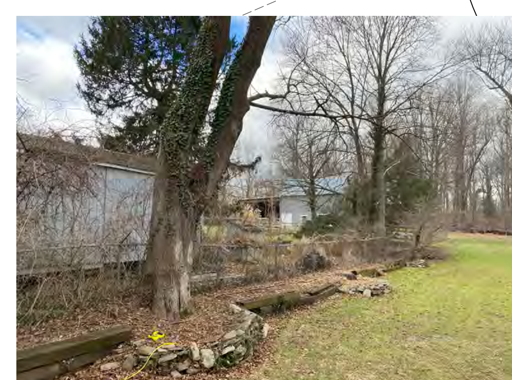
View of Existing Timber Retaining Wall to be Replaced Existing Stone wall to be removed + Feather out the Grade
