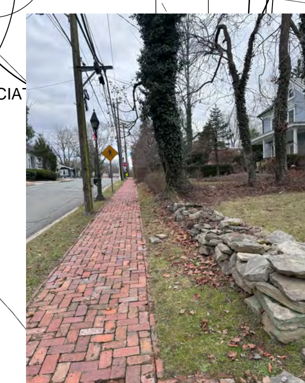
Existing Retaining Stone Wall and Public Side Walk
