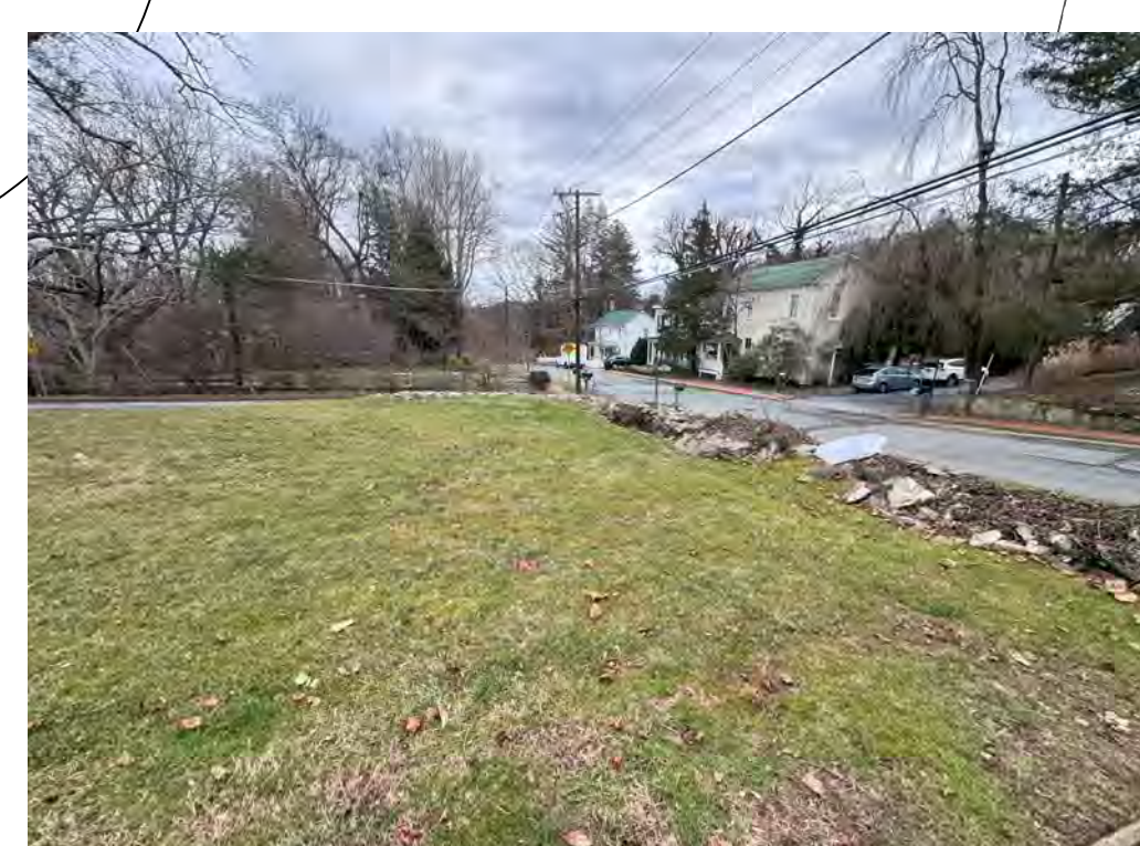
View of Existing Stone Wall to be Re-Stacked - Wall width to be between 24" to 30"
