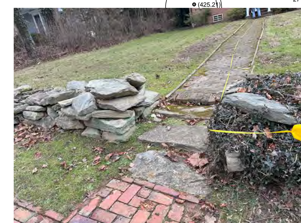
Existing Stone Wall to be Re-stacked and Reset Top Brick Step and/or Stone Step = TBD onsite w/ Mason
