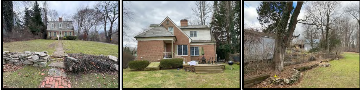
Figure 3: The applicant provided these photos of the existing property that show the front elevation, rear elevation, and retaining wall at the south property line.
