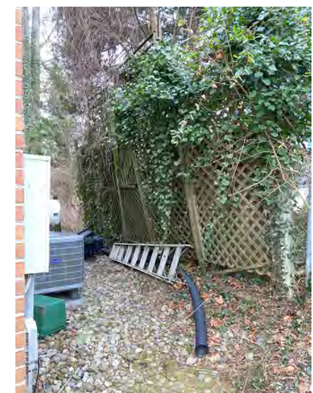
Existing Lattice Screen to be Removed
