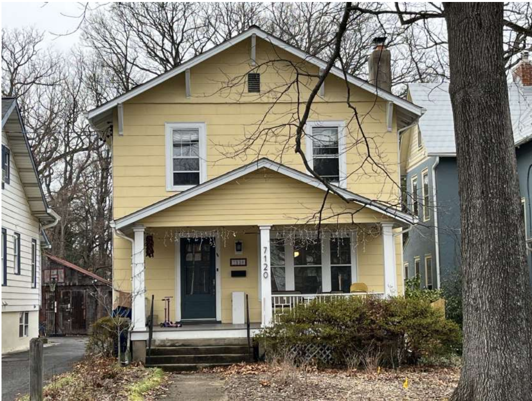
Detail: 7120 MAPLE AVE. FRONT
