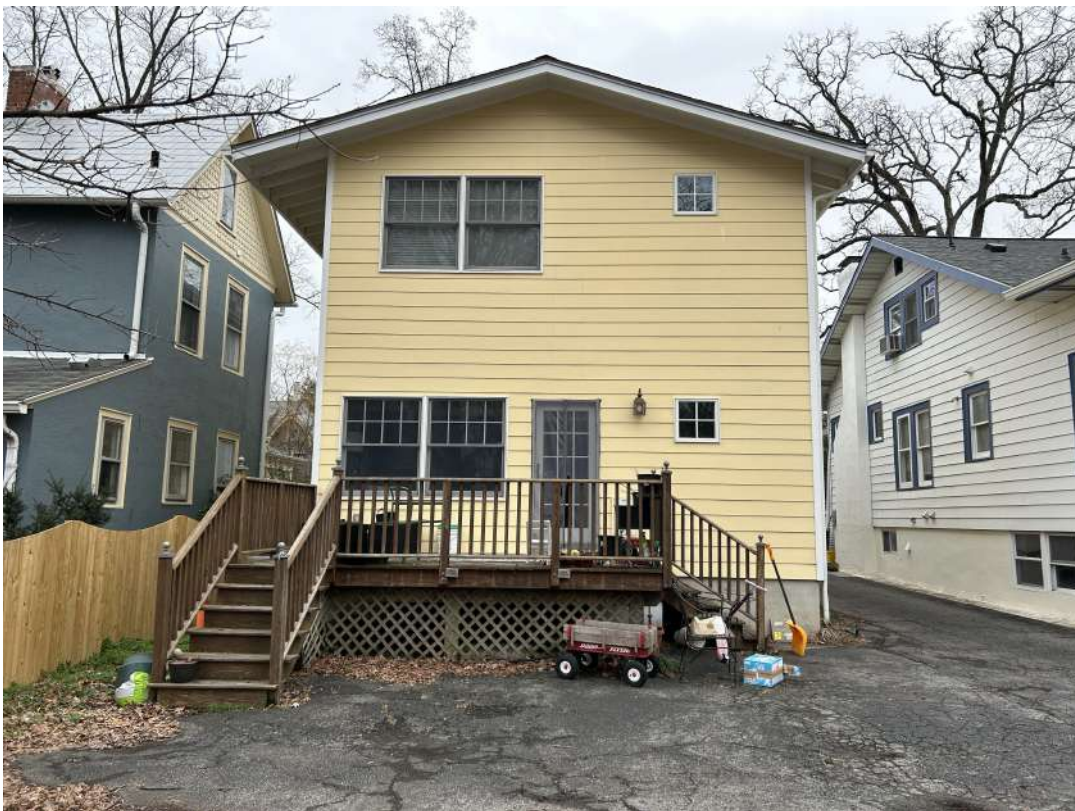
Detail: 7120 MAPLE AVE. REAR
