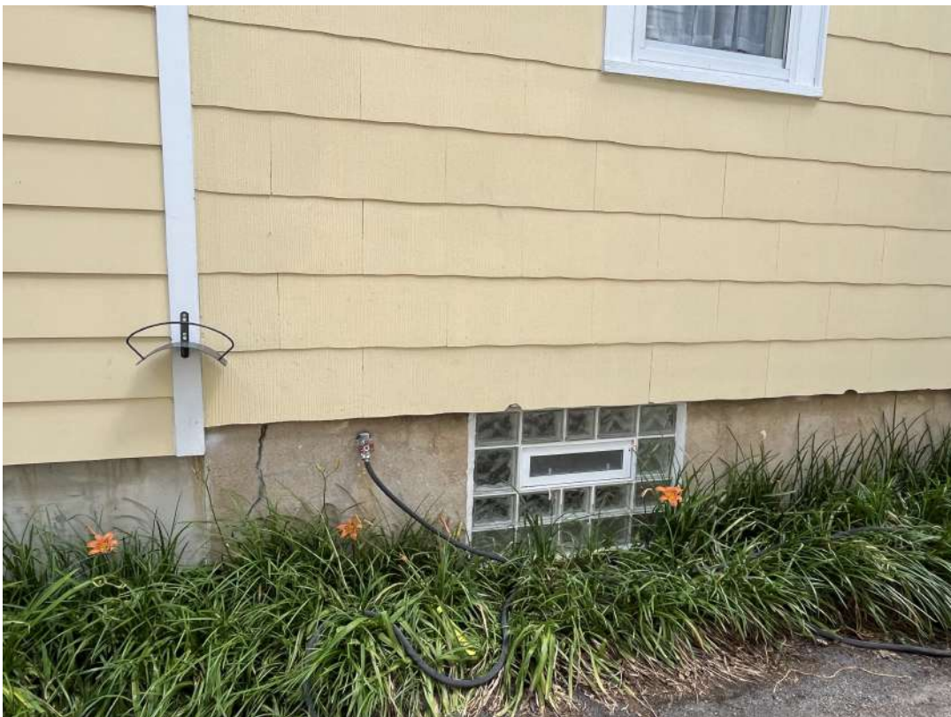
Detail: 7120 MAPLE AVE. BASEMENT WINDOW & SIDING
