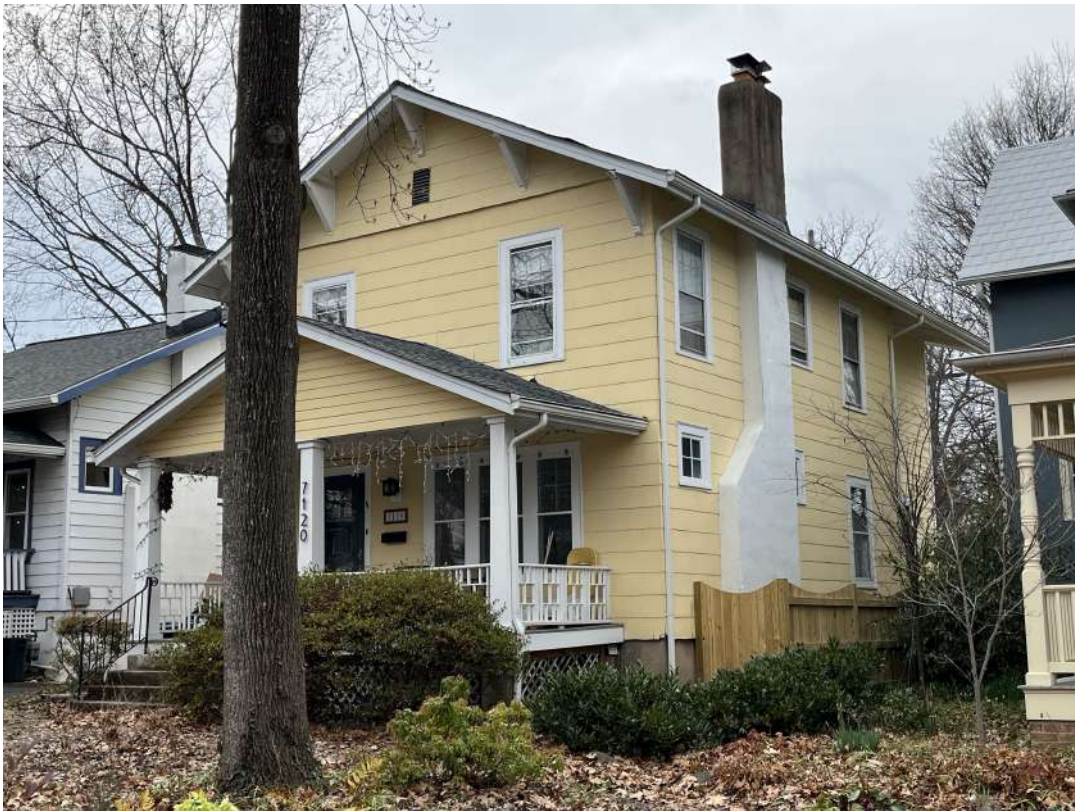
Detail: 7120 MAPLE AVE. NORTH-EAST APPROACH
