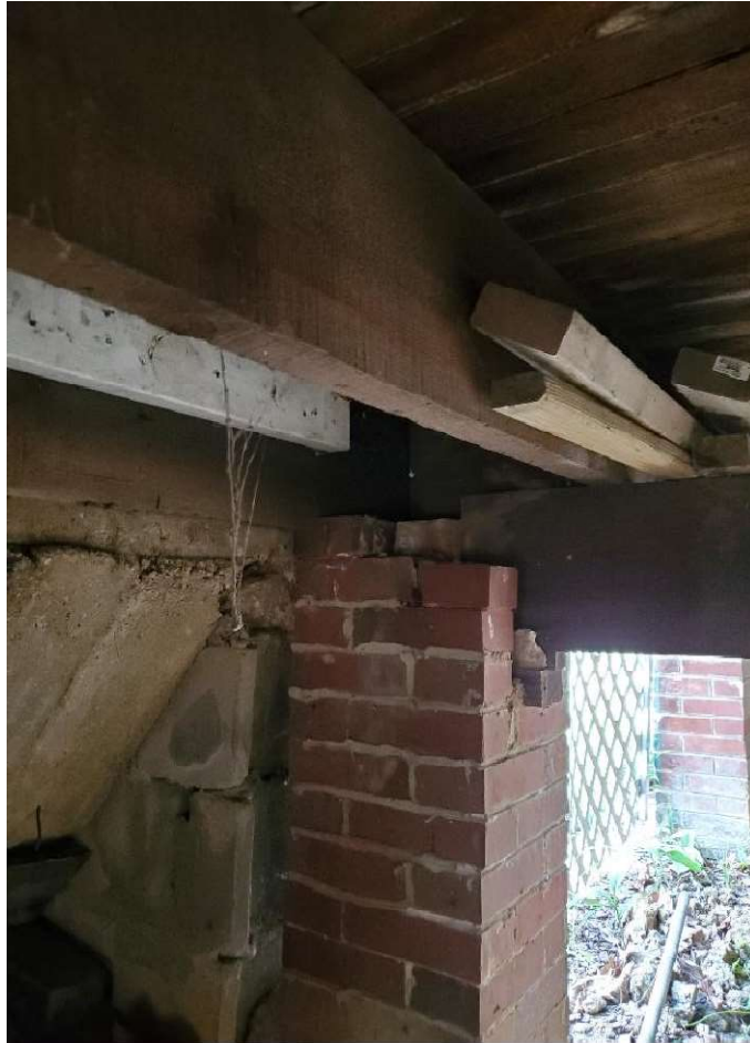
Photo 18 - 7102 Maple Ave – brick pier
