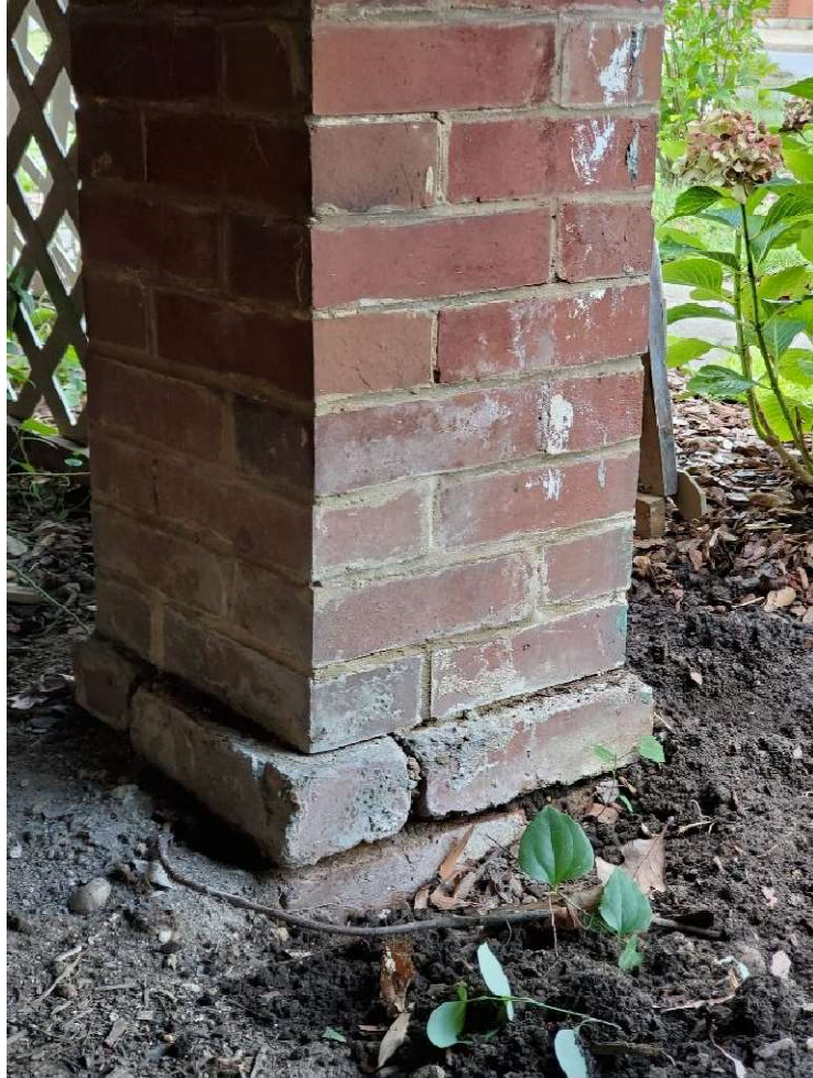
Photo 13 - 7102 Maple Ave – brick pier base
