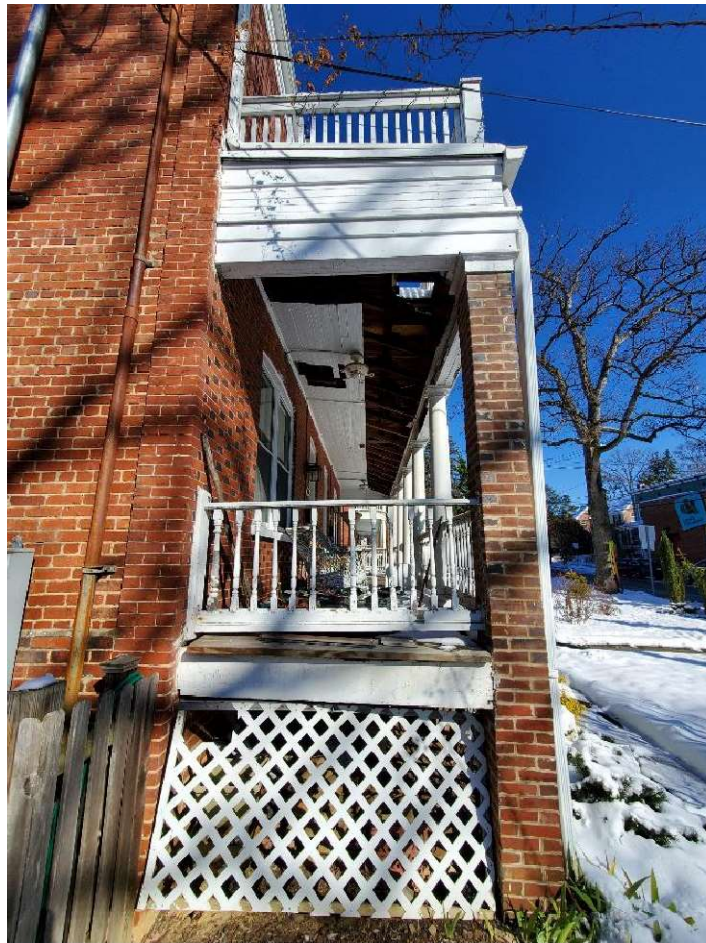
Photo C - 7102 Maple Ave – Side Elevation-South
