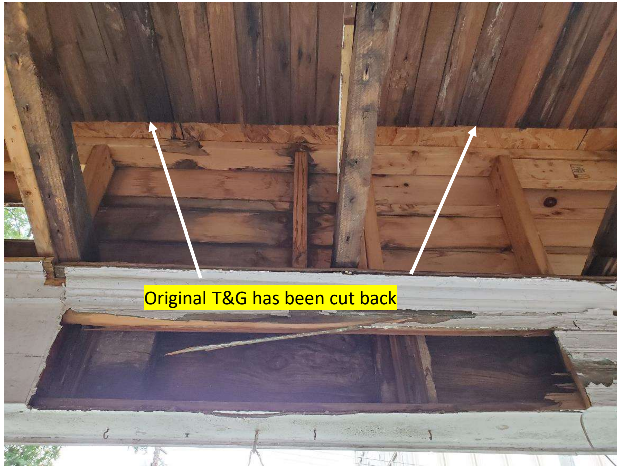
Photo 16 - 7102 Maple Ave – ‘wall’ above support beam
