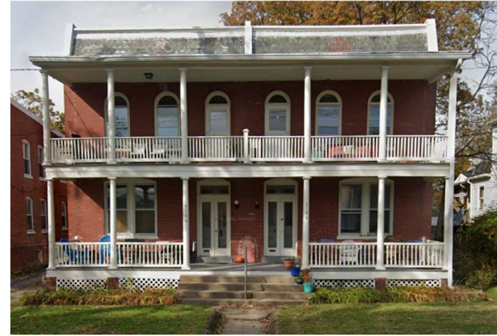
7106-8 Maple Ave – Fascia
