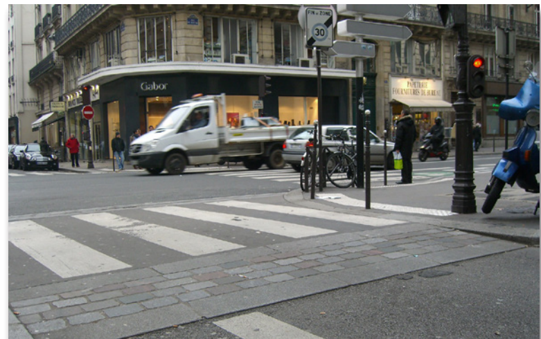
A raised crossing at sidewalk level across a low-speed, low-volume street. Photo Credit: Vladimir Zlokazov
