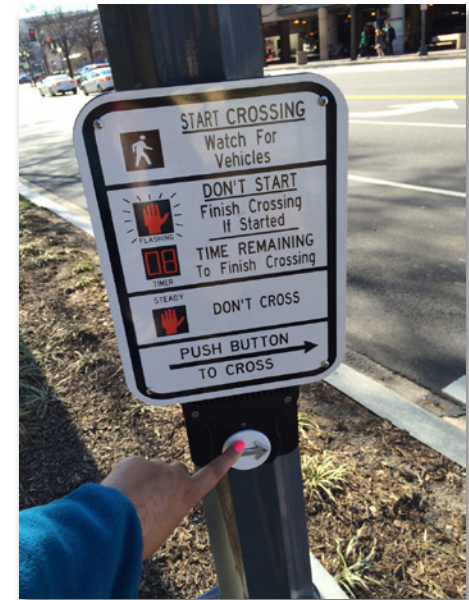
A pedestrian push button. Photo Credit: Montgomery County Government
