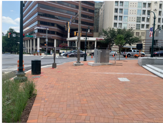
Traffic signal control cabinet in the sidewalk in downtown Silver Spring
