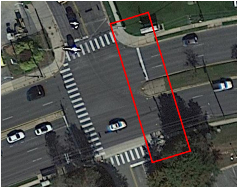
With the crossing in the red box missing, pedestrians must use the other three crosswalks to get between the upper and lower corners on the right side. Image Credit: Google Maps
