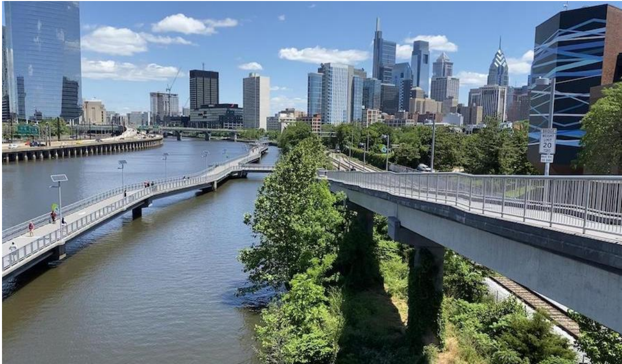
Figure 5.6: Schuylkill River Trail, located adjacent to University City District
