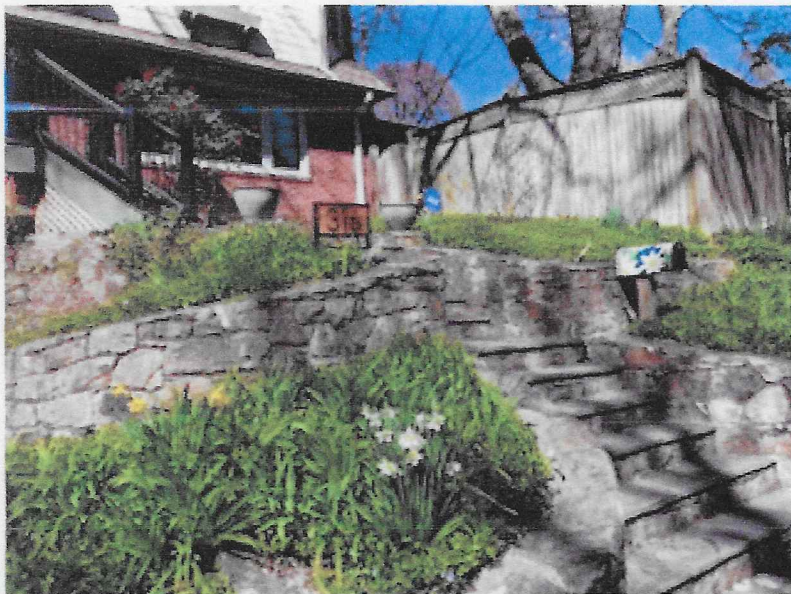
316 Elm Avenue corner lot with high fence for portion of yard.
