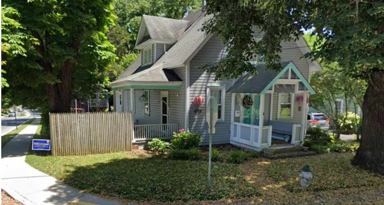
Figure 2: The existing stockade fence engages the northwest porch column.
