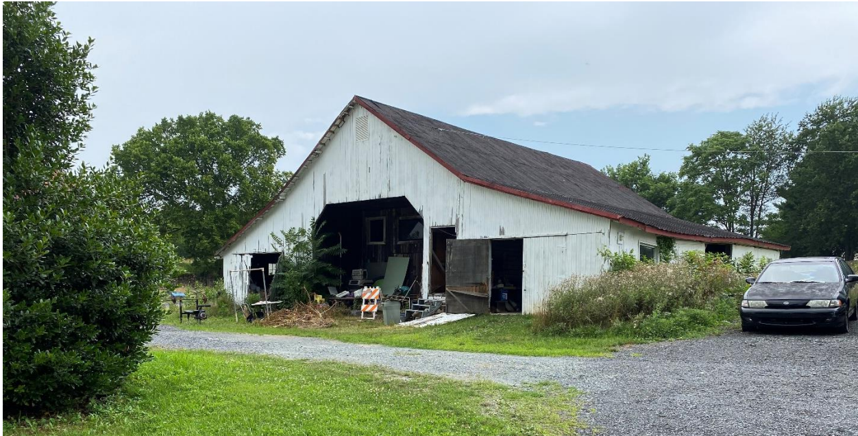
Figure 3: Staff photo of the barn.
