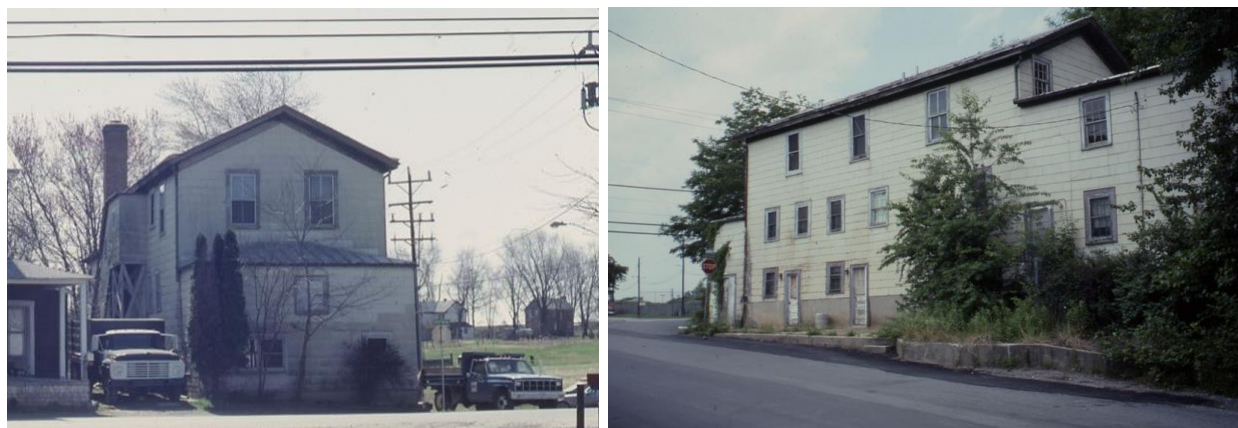
Figure 2: File photo (c.1980) showing the window placement and window type.
