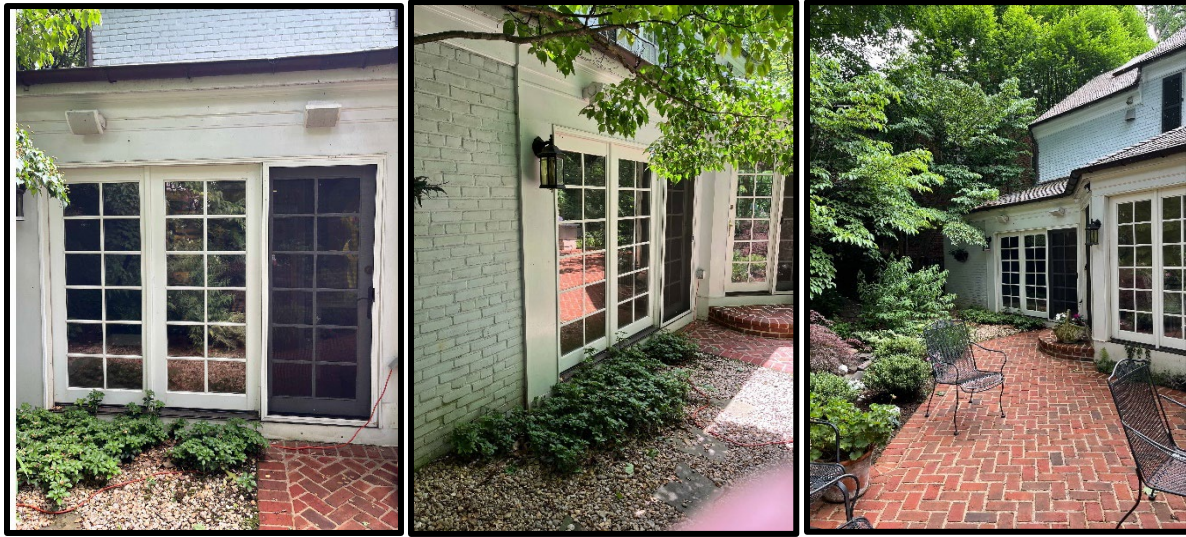
Figure 2: The existing triple doors on the rear elevation to be removed and replaced with French doors.
