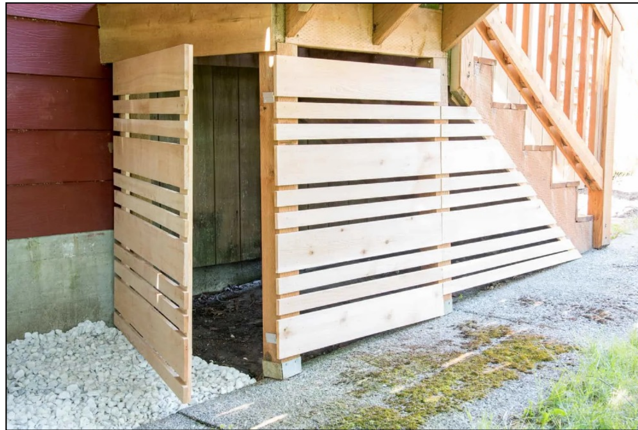
Hinged under deck facing to allow for storage
