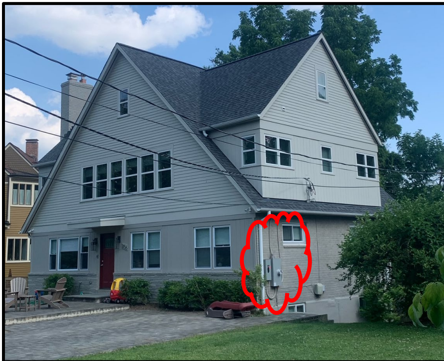
Figure 5: Some of the panels' equipment will be installed on the west elevation near the existing electrical meter in the area clouded in red.
