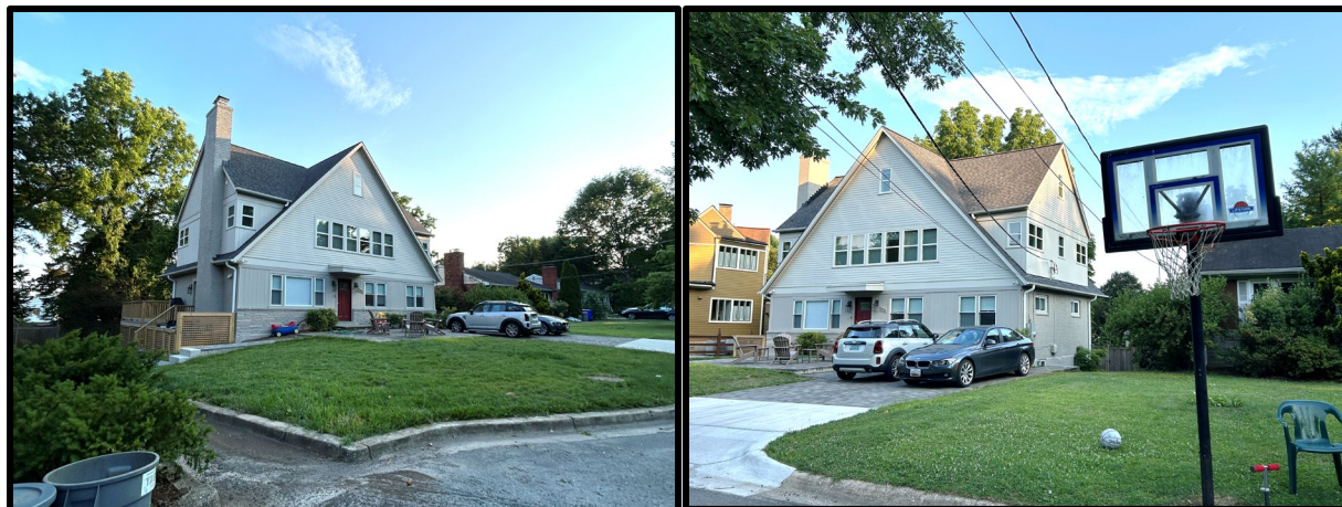
Figure 2: The front and left-side elevations, left, and the front and right-side elevations, right.
