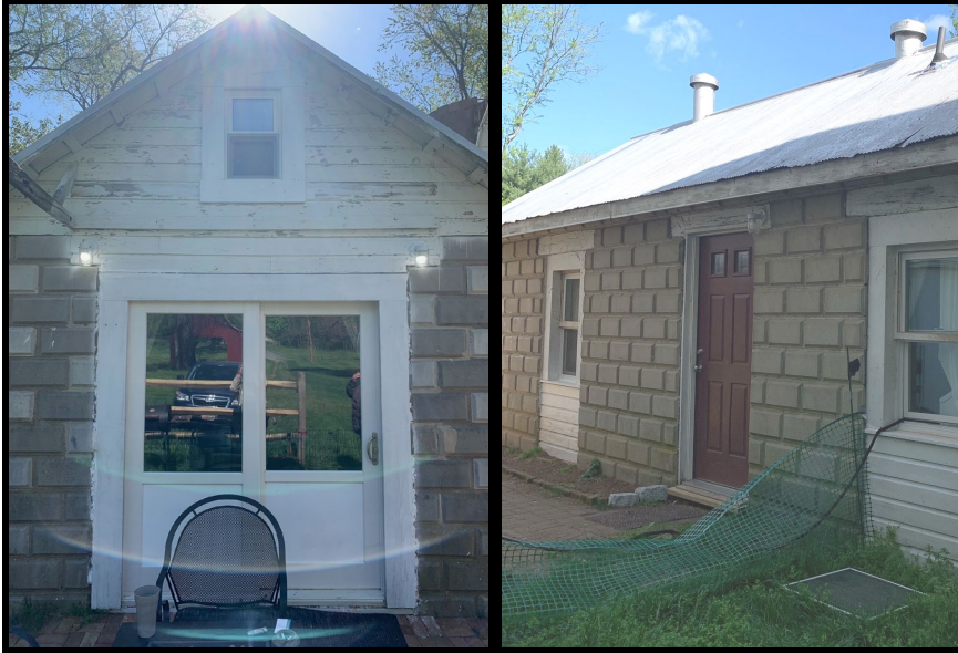
Figure 12: The sliding composite doors on the front elevation, left, and the fiberglass door on the right-side elevation. The lights are circled in red.
