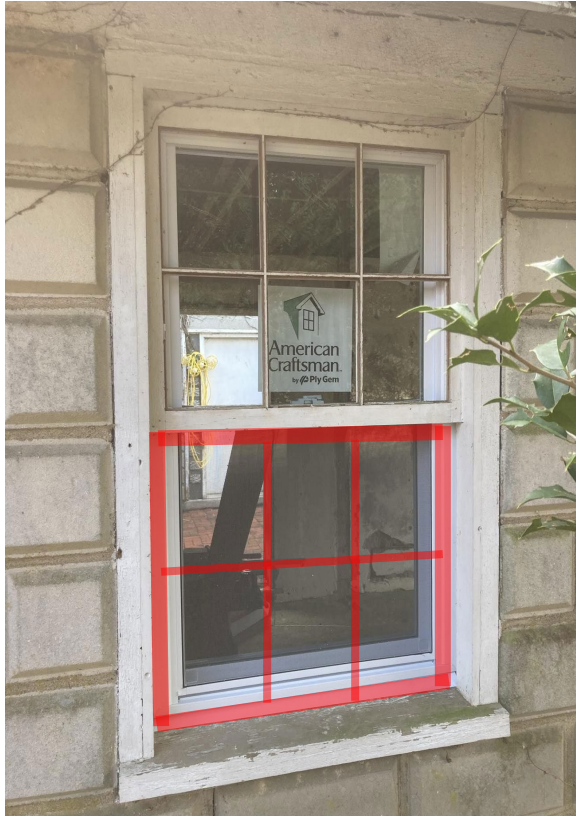
Replacement of one (1x) six over six lower wooden window sashes
