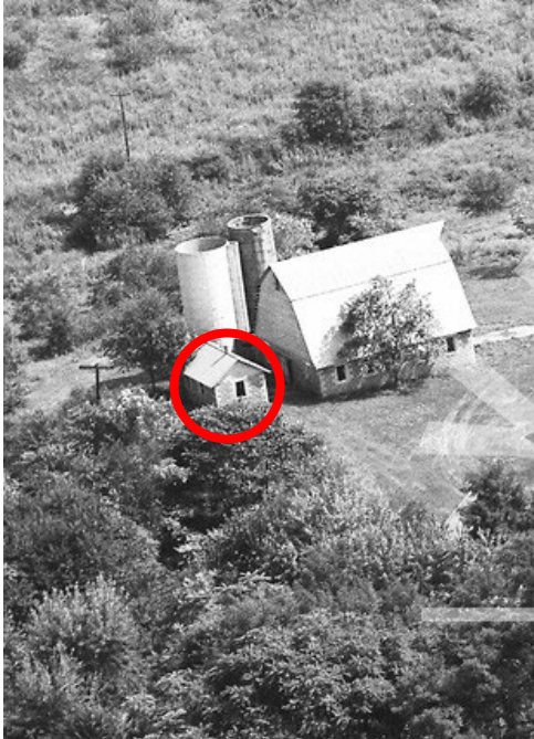
Figure 4: This cropped Vintage Aerial photo from 1973 show the Milk House before the façade was altered.
