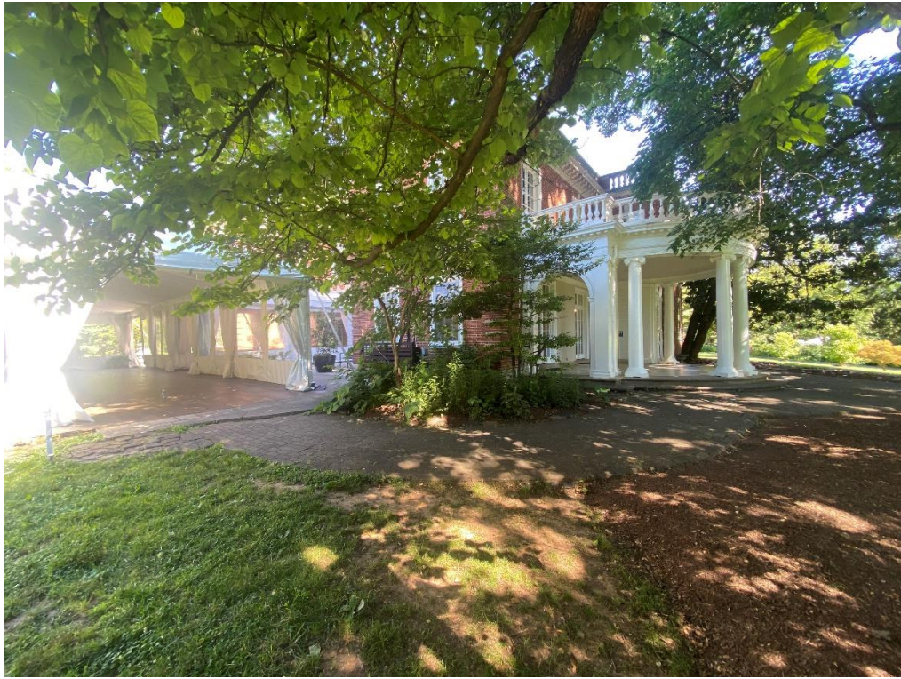
Woodend: East walkway from terrace to portico
