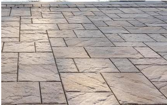
Proposed Terrace Paver: TechnoBloc Slate-faced Blu60 pavers Pattern to match existing
