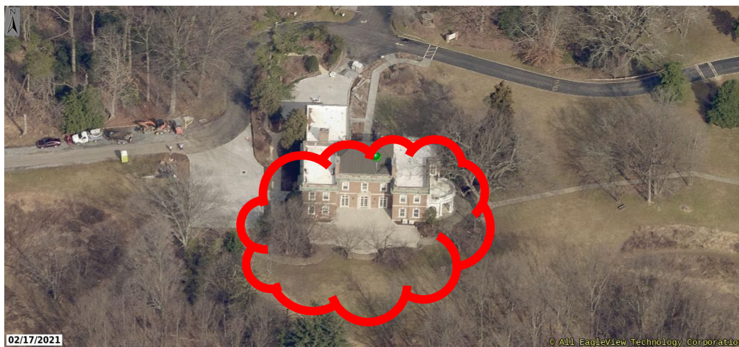
Figure 2: The concrete paver terrace behind the Woodend Mansion is clouded in red. Source: CONNECTExplorer
