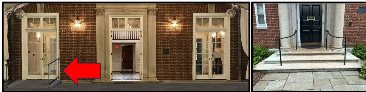
Figure 4: The applicant provided this rendering to show the proposed handrails and ramp at the rear of the mansion, left. The handrails will be similar in appearance to those found at the west entrance to the mansion, right.
