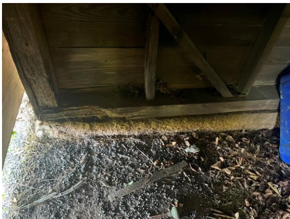
View of partition wall separating south and north bays, view from south bay looking north. Note studs on interior of south bay and cladding on side facing the north bay, and the concrete foundation (similar to rear (west) and side (south) walls in this bay, but not present in the north bay).
