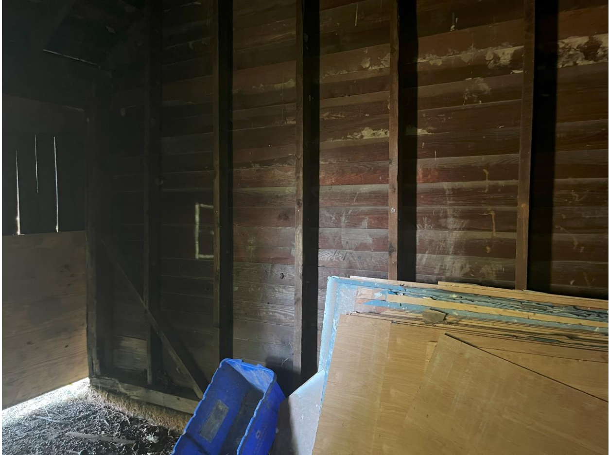
View of partition wall separating south and north bays, view from south bay looking north. Note studs on interior of south bay and cladding on side facing the north bay, and the concrete foundation (similar to rear (west) and side (south) walls in this bay, but not present in the north bay).
