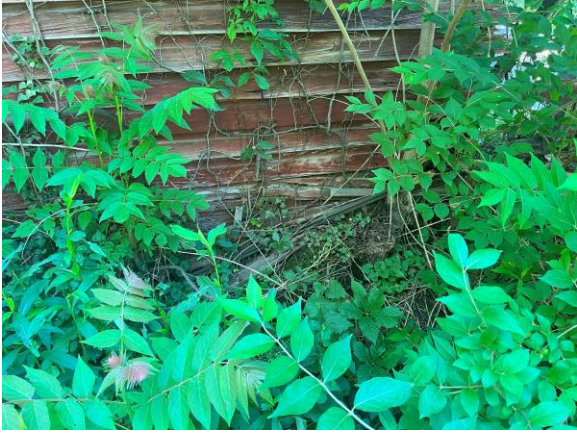
Details of siding and north bay barn doors.
