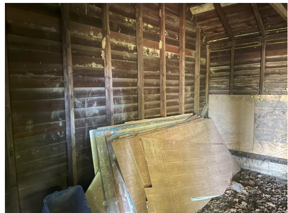
View of partition wall separating south and north bays, view from south bay looking north. Note studs on interior of south bay and cladding on side facing the north bay, and the concrete foundation (similar to rear (west) and side (south) walls in this bay, but not present in the north bay).
