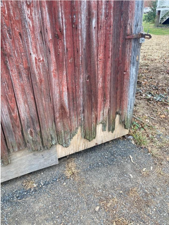
Details of deteriorated condition of shed.
