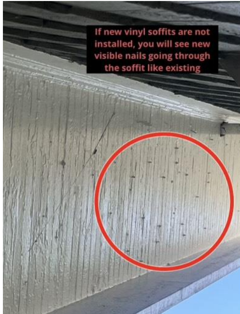
Figure 3: Photo of the existing soffits, provided by the applicant.
