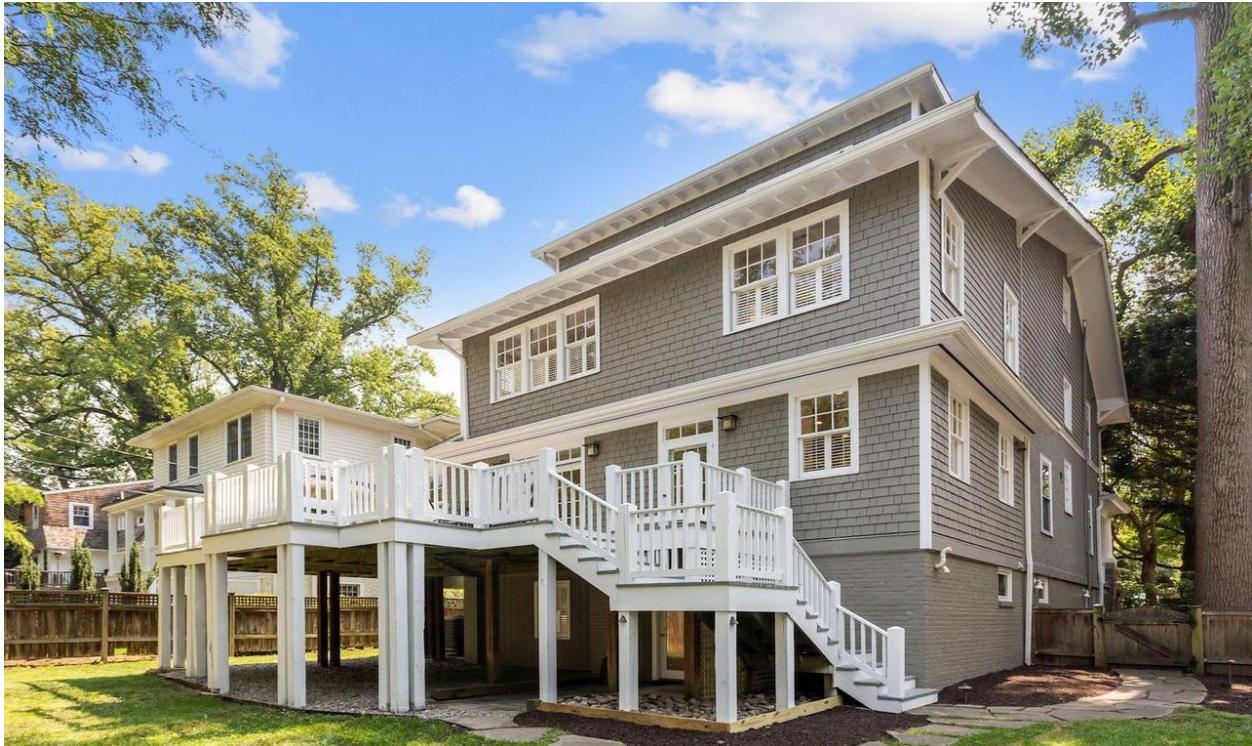
Figure 2: Photo of the rear of the house before the soffits were boxed in.
