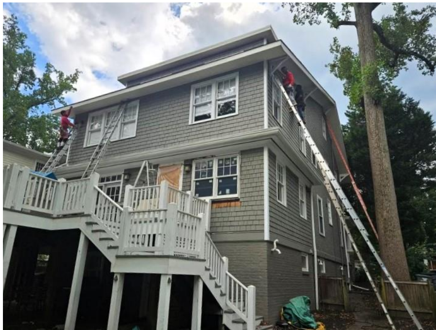
Figure 4: Rear of the house after the soffit had been boxed in.
