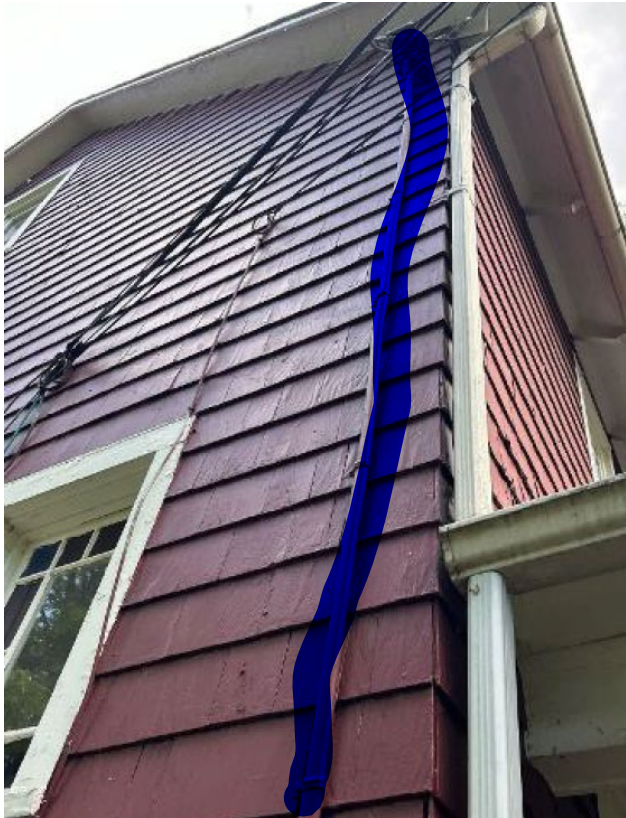
Utility Meter After
