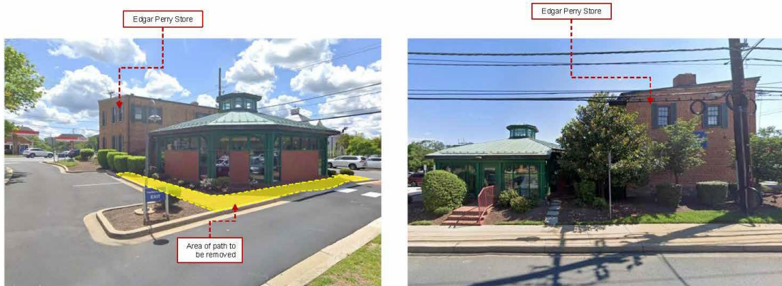
Figure 2: The Perry Store facing southeast, left, and facing north, right.
