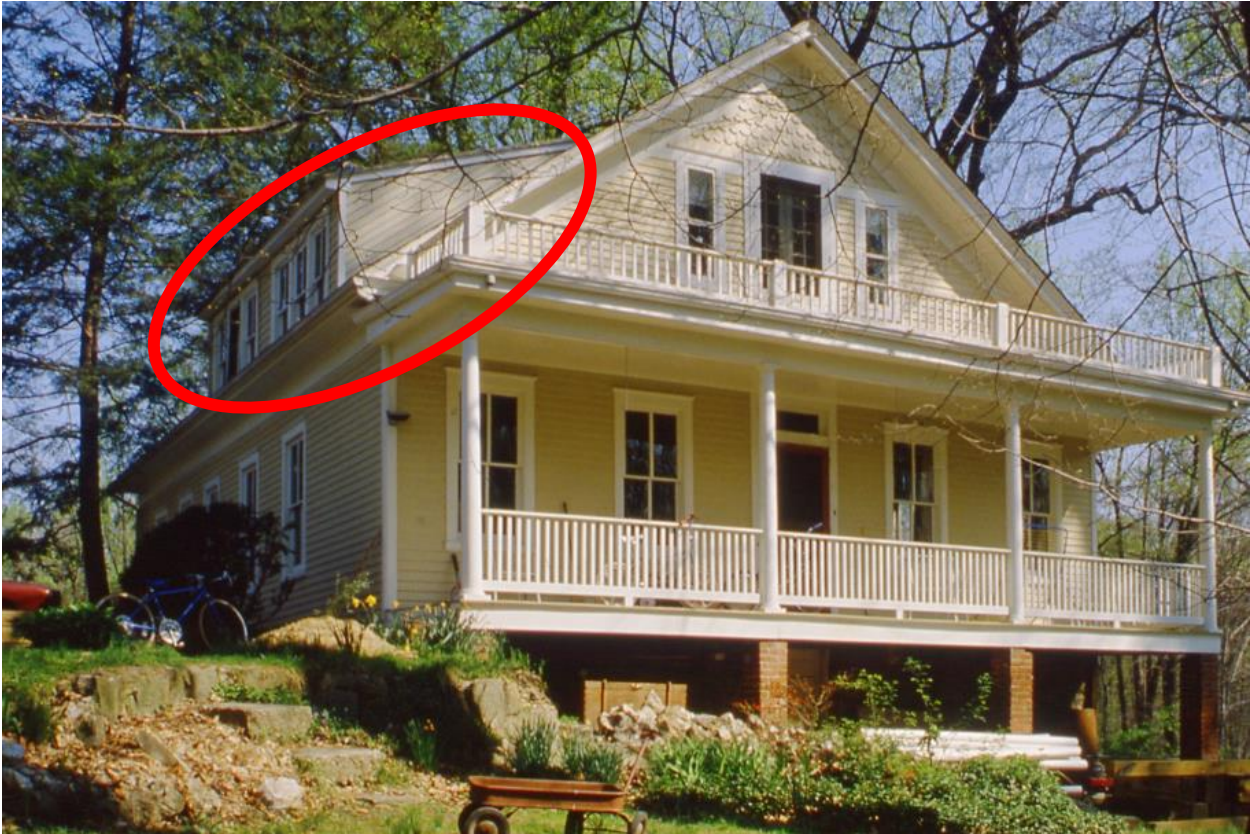
Figure 4: HP file photograph of the subject property before the siding replacement.
