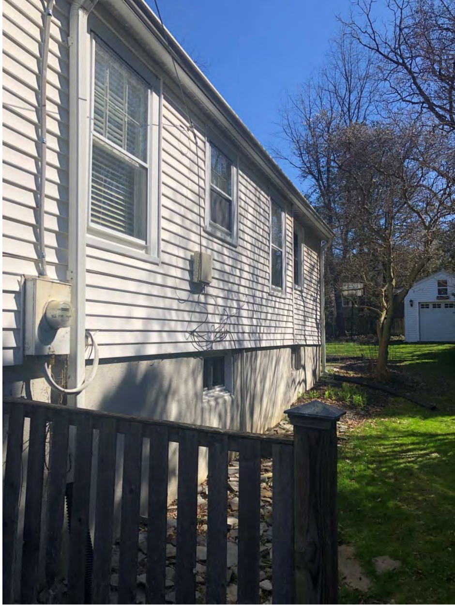
SOUTH FACADE WITH VIEW OF TREE TO BE REMOVED. SEE DRAINAGE NOTE BELOW
