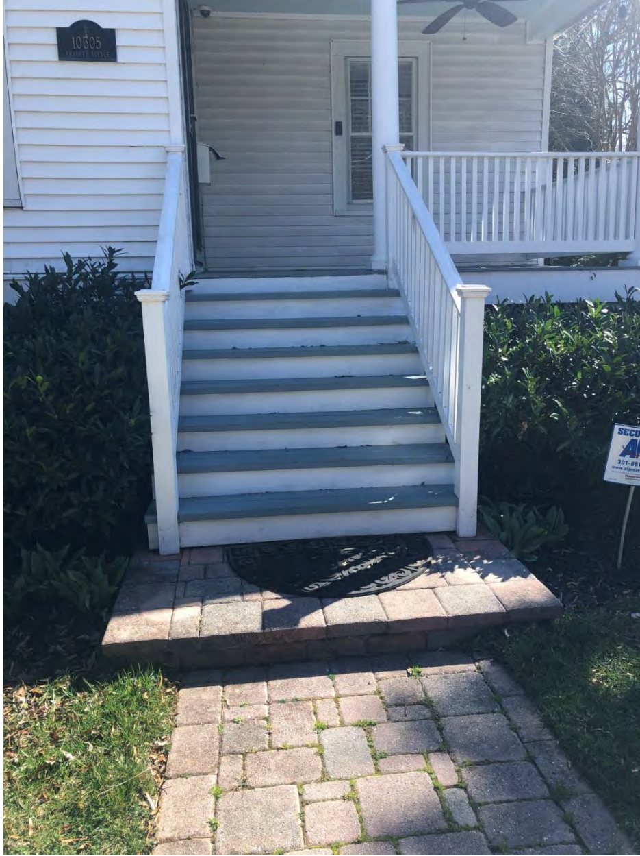
CLOSE UP SHOT OF FRONT STAIRS...RAILING REMAINS , PAVERS REMAIN. STAIR TREADS PROPOSED WITH NEW TREX REPLACEMENT (MAY REQUIRE RESTRUCTURING STAIR UNDERNEATH)
