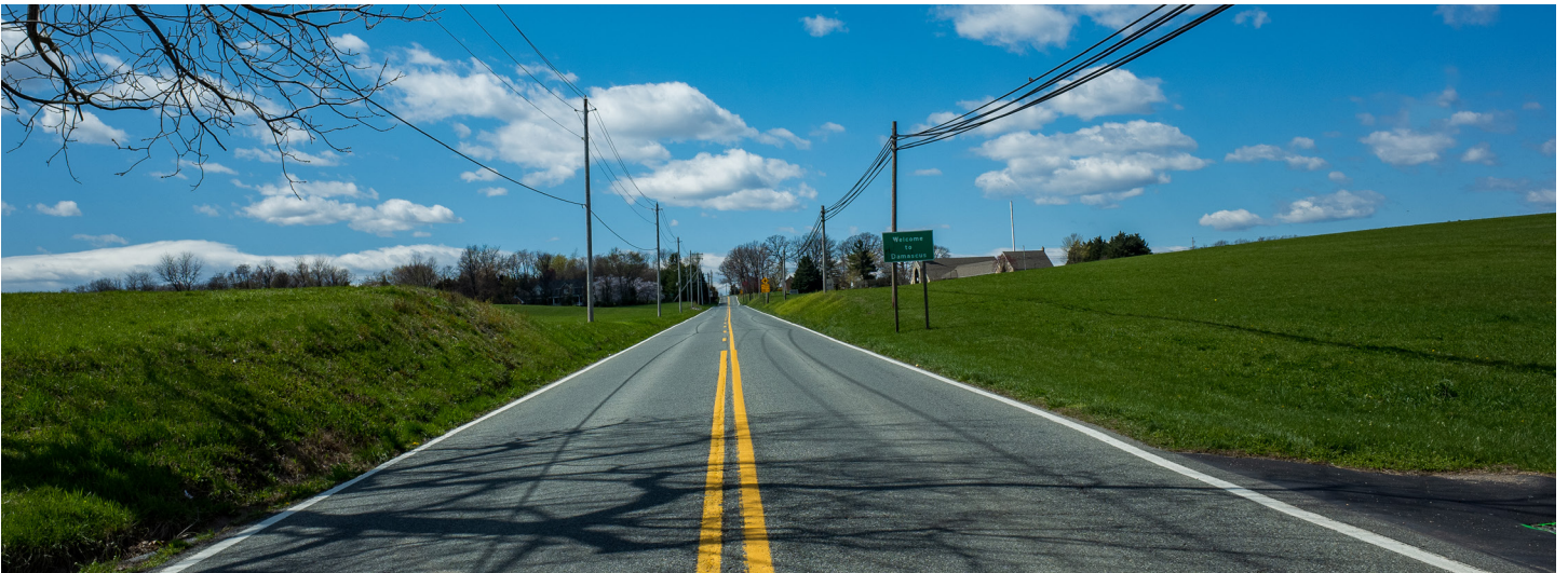
Figure 2-87. New Hampshire Avenue / Damascus Road (MD 650) between Ashton and Damascus
