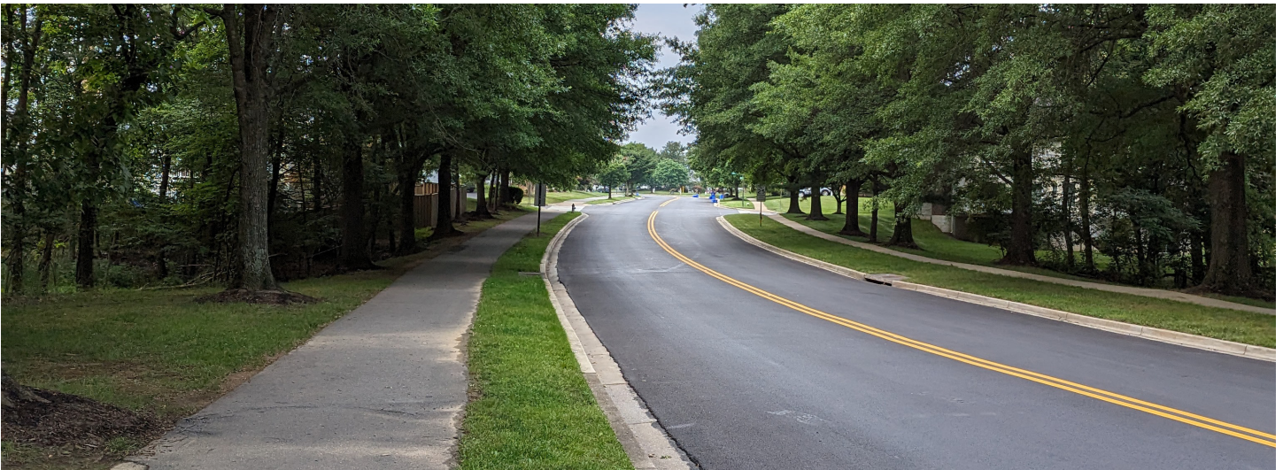
Figure 2-59. Stonebridge View Drive between Muddy Branch Road and Travilah Road
