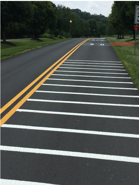
Figure 8-11. Example of optical speed bars
