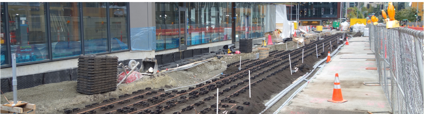
Figure 7-5. Soil cells being installed to provide structure under a future sidewalk.
