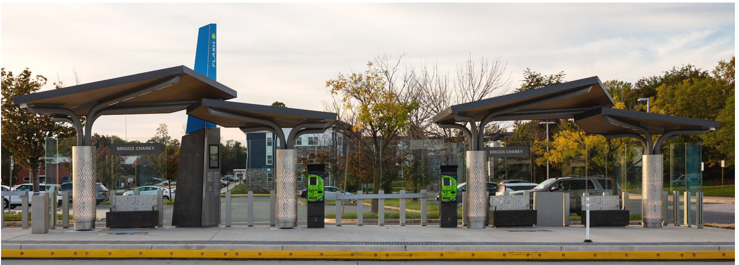
Figure 3-20. Briggs Chaney BRT station
