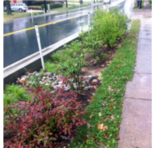
Figure 7-7. Examples of rain gardens (Source: Montgomery County Department of Environmental Protection)
