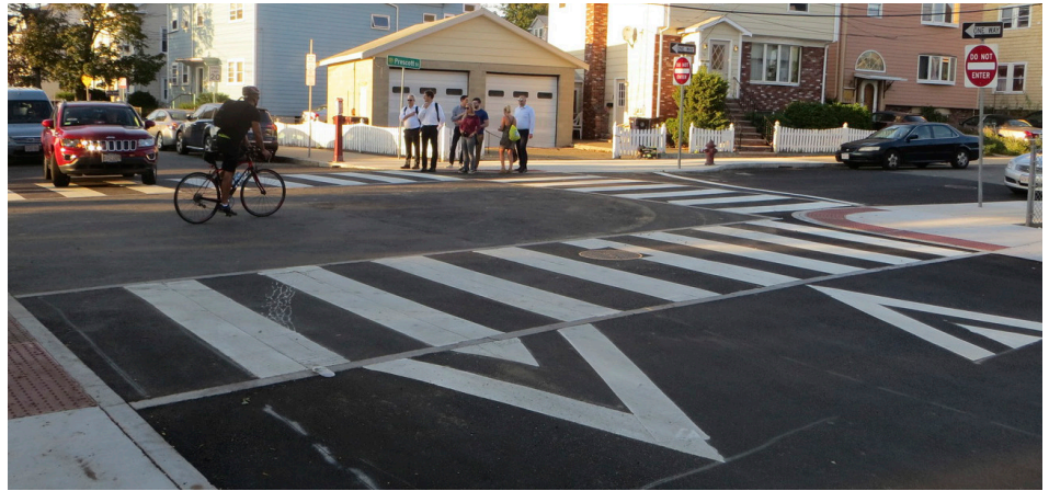
Figure 6-35. Image of a raised intersection
