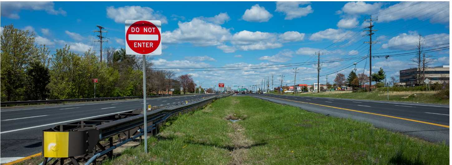
Figure 2-101. Columbia Pike (US Route 29) from Prelude Drive to the Howard County Line
