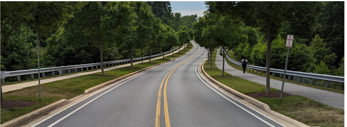
Figure 2-51. Foreman Blvd between Snowden Farm Parkway and MD 355
