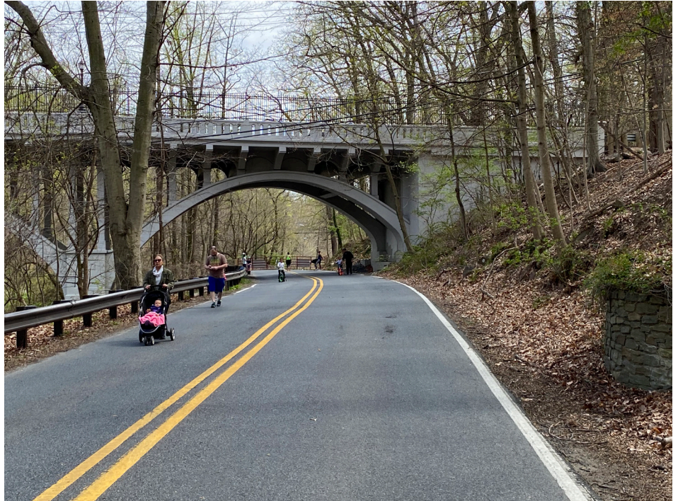
Figure 2-109. Closed Sligo Creek Parkway under Carroll Avenue Bridge
