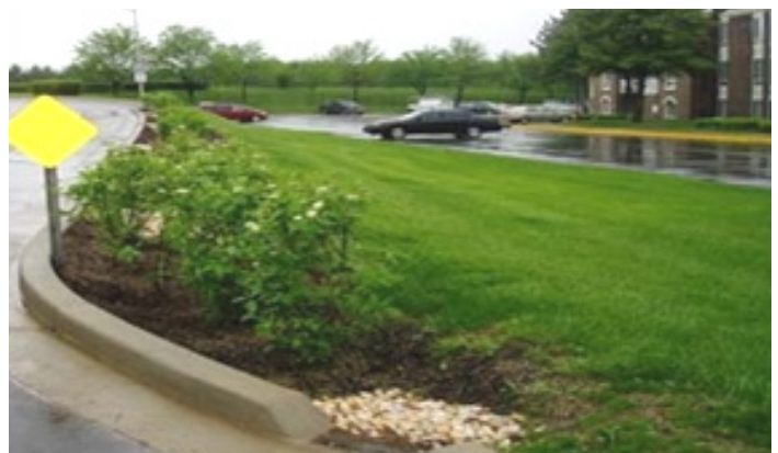
Figure 7-9. Examples of green infrastructure treatments in Montgomery County
