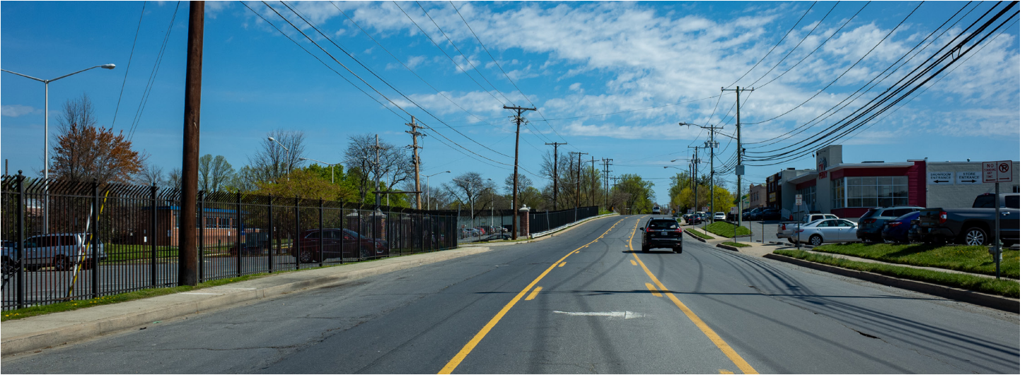
Figure 2-78. Brookville Road in Lyttonsville
