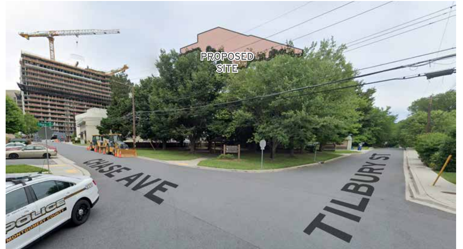
VIEW LOOKING WEST ON HIGHLAND AVE
