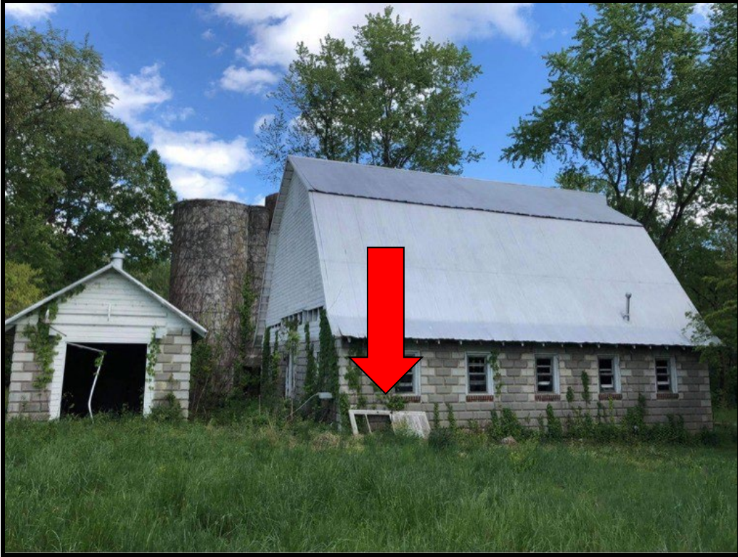
Figure 15: The applicant provided this circa 2021 photo of the Milk House and Dairy Barn. The arrow points to what appears to be a wood screened door that may have been installed on the Milk House or Dairy Barn.
