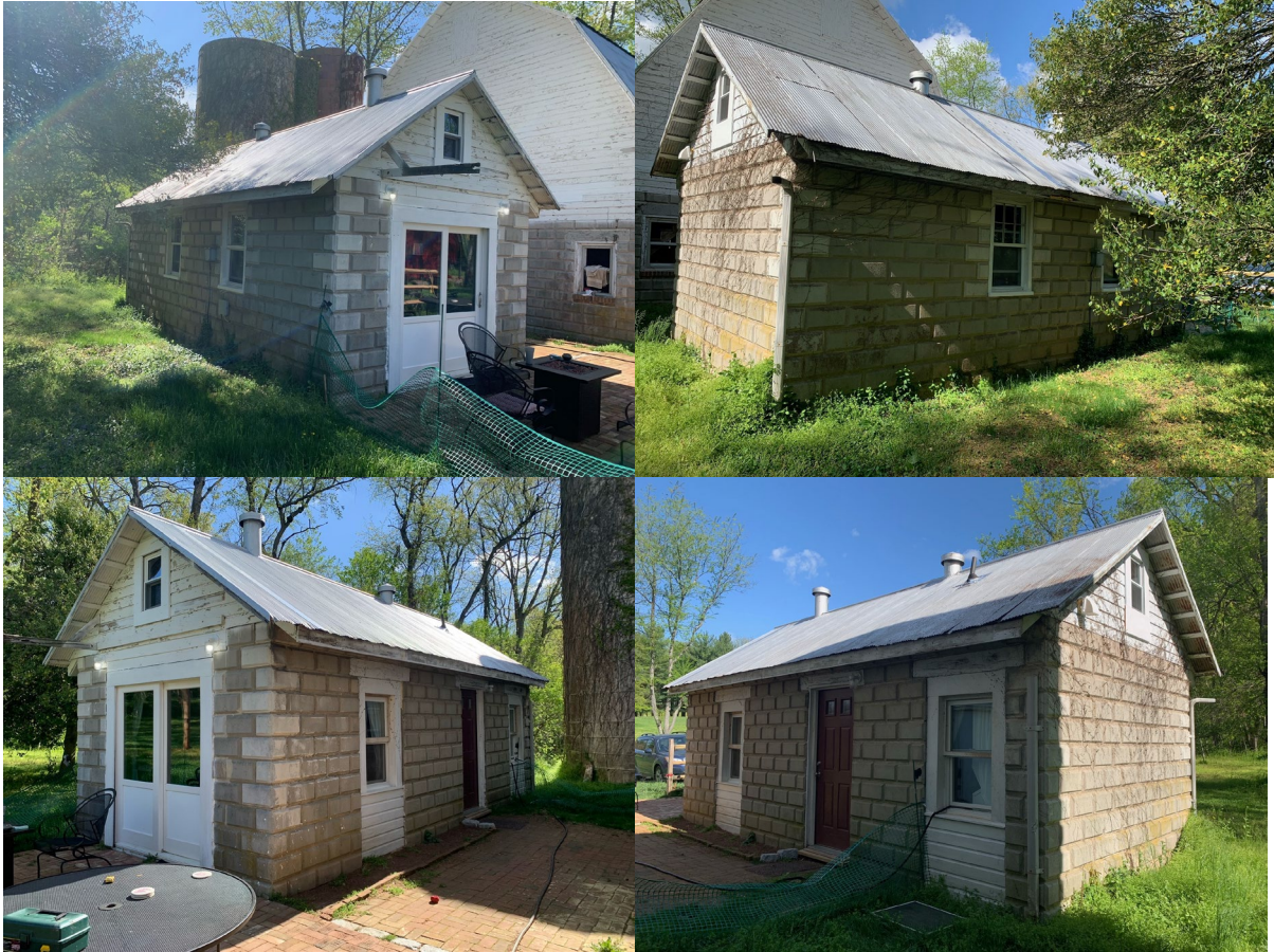
Figure 3: Clockwise from top left: front and left-side elevations; left and rear elevations; rear and right elevations; and right and front elevations.
