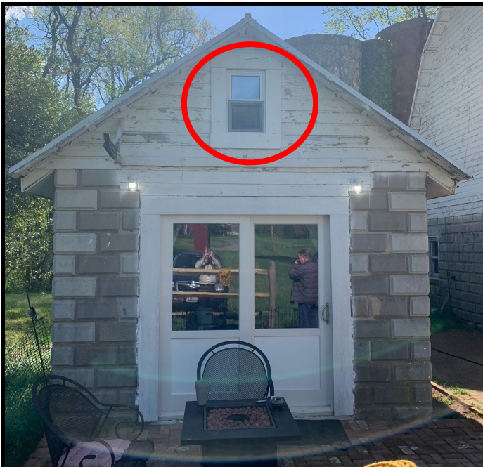
Figure 16: The trim around the new front gable end opening.
