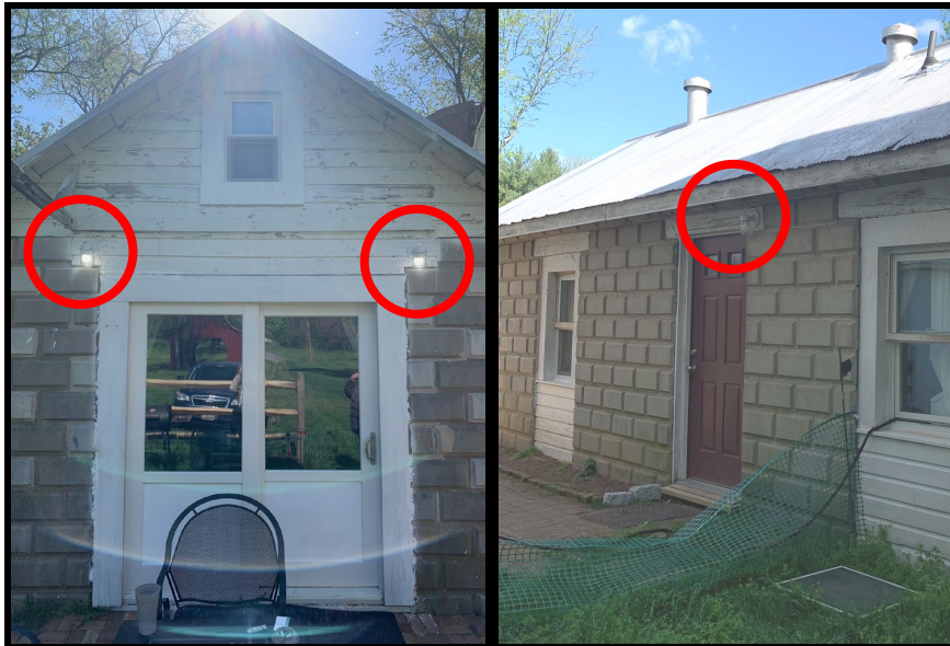
Figure 10: The sliding composite doors on the front elevation, left, and the fiberglass door on the right-side elevation. The lights are circled in red.
