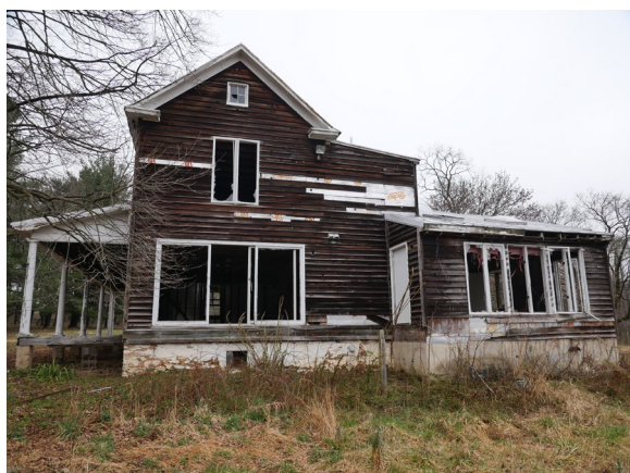
Figure 10: The rear elevation in 2021 and the proposed. The applicant proposes to demolish the existing shed-roofed addition and build a new two-story addition in its place, outlined in red. He also proposed fenestration alterations on the portion of the building to be retained.
