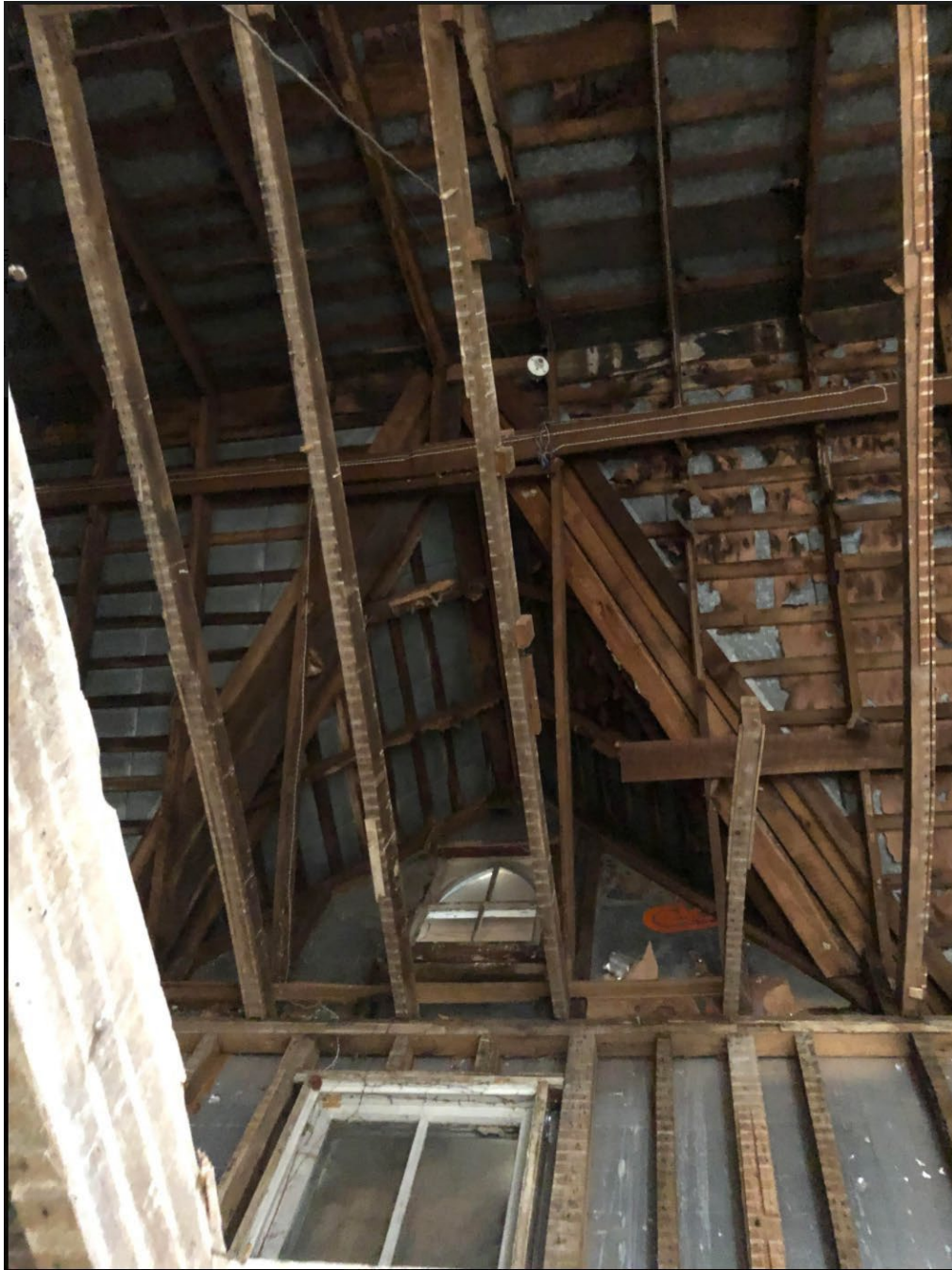
Interior Main Gable and Front Dormer
