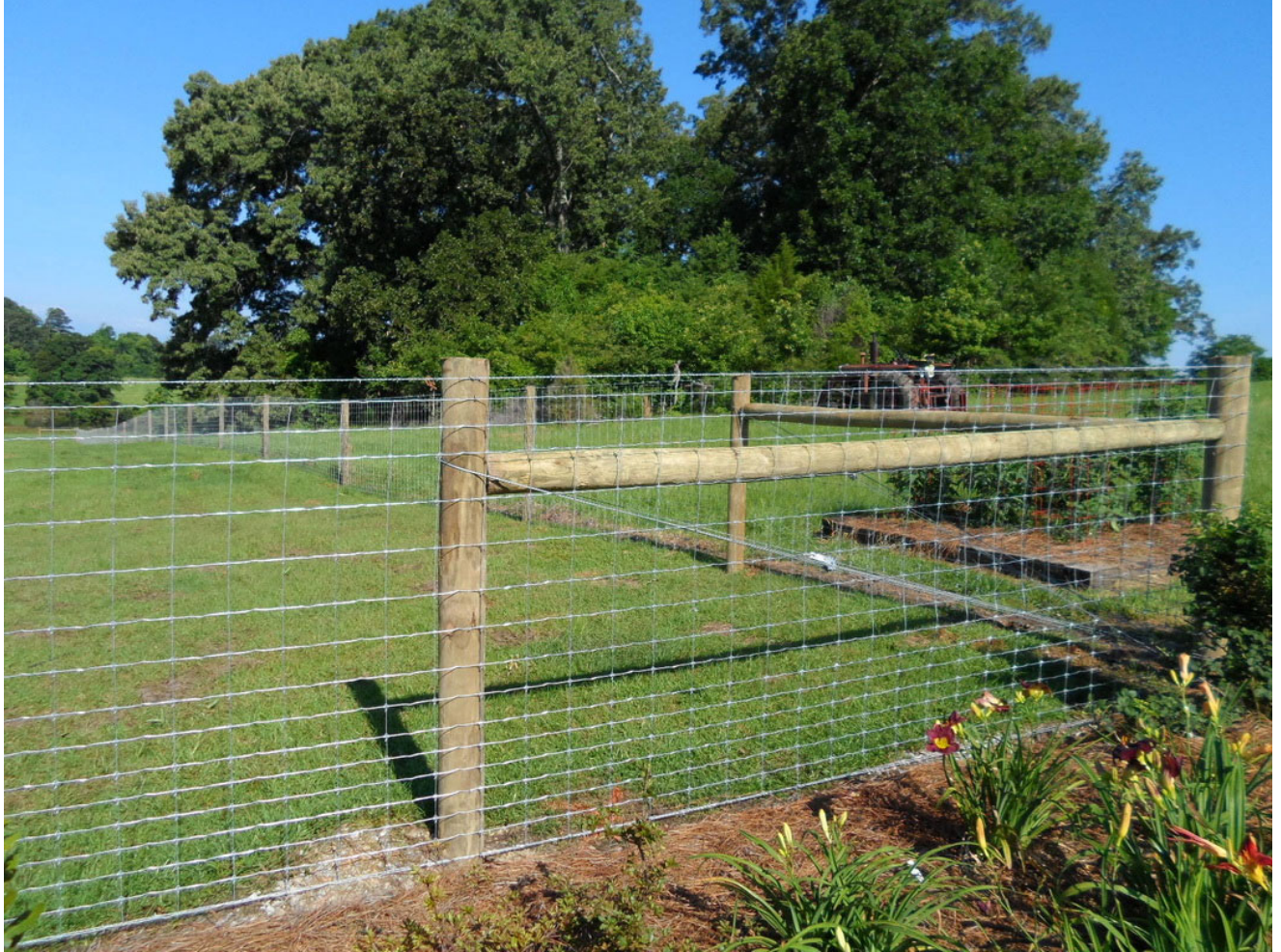
Sample woven wire fence with pressure treated wood posts
