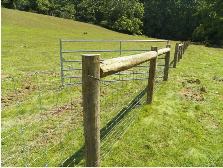
Figure 4: The applicant proposes to install a wood post and wire fence with metal gates.
