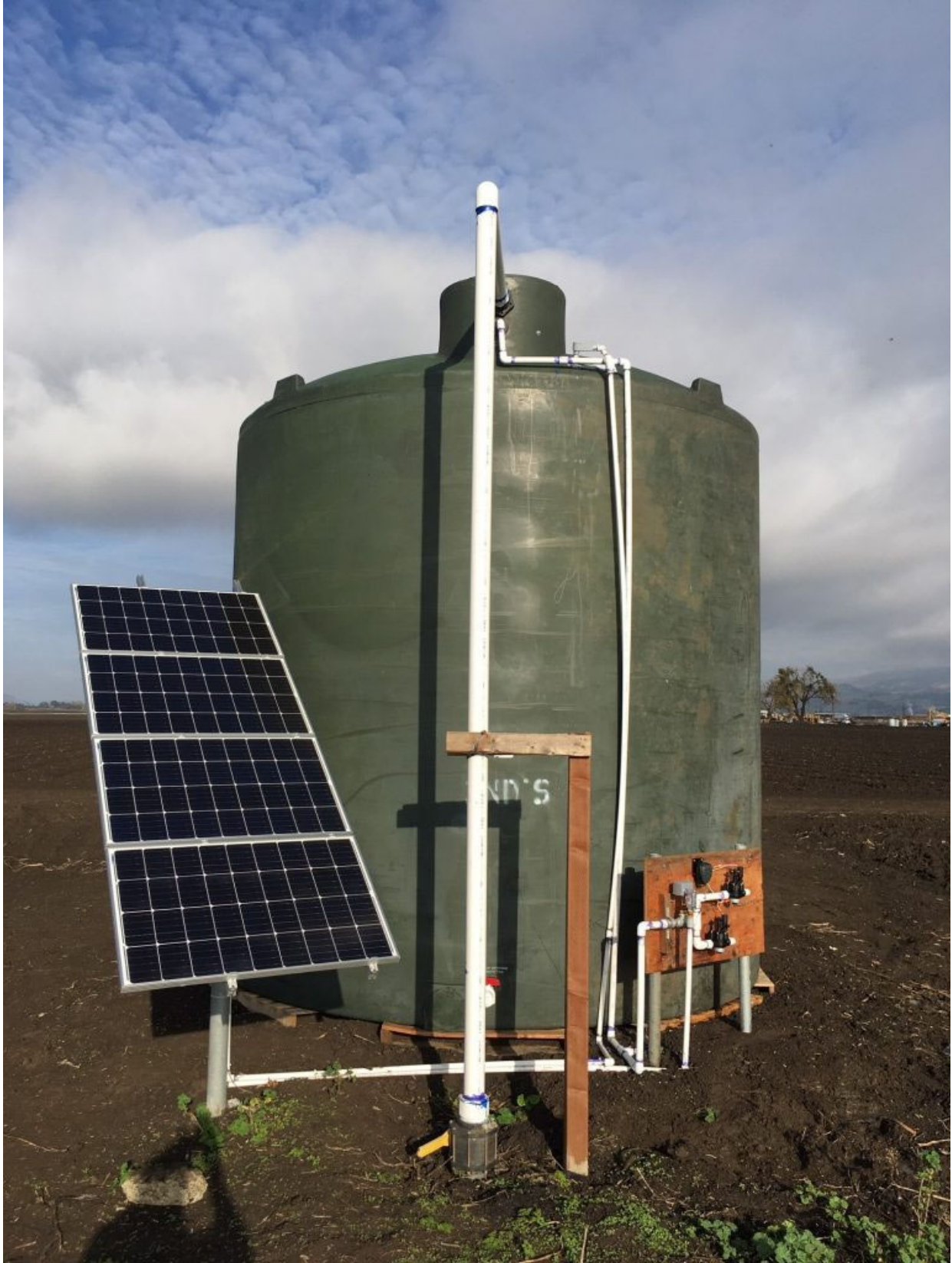
Sample photo of solar charger and above ground plastic water storage tank
