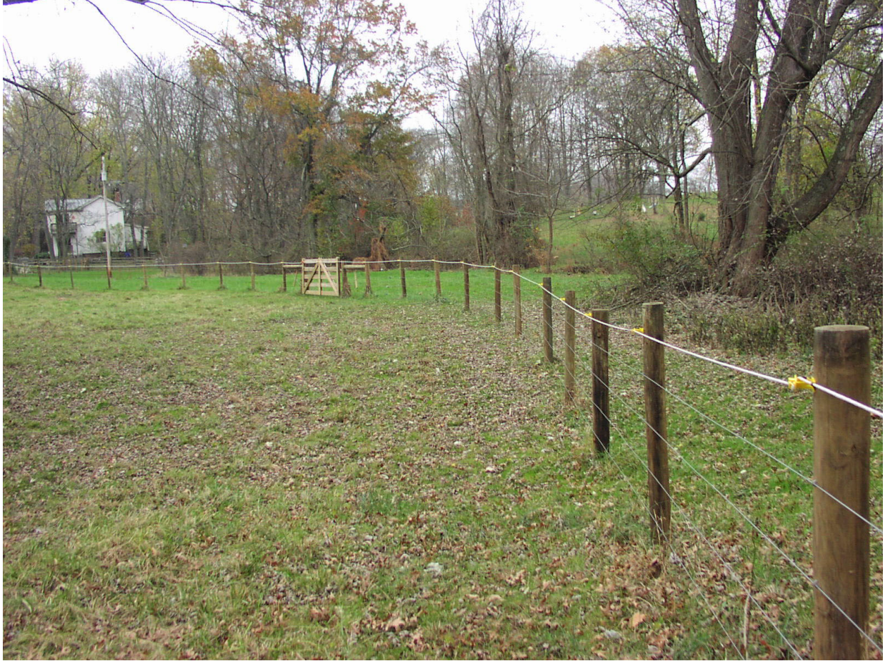
High Tensile Wire with Wood Posts
