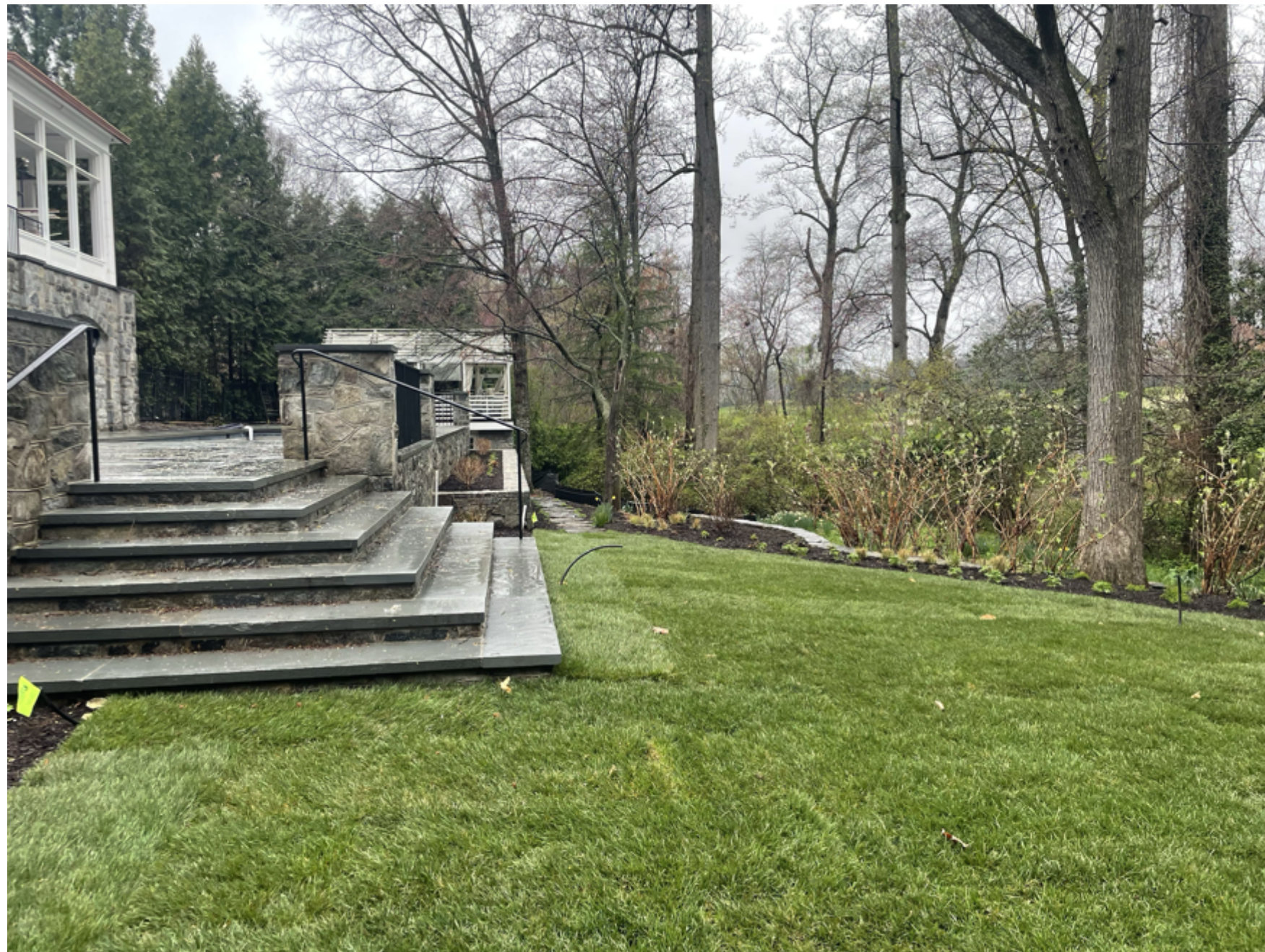
EXISTING STAIRS TO LOWER LAWN
