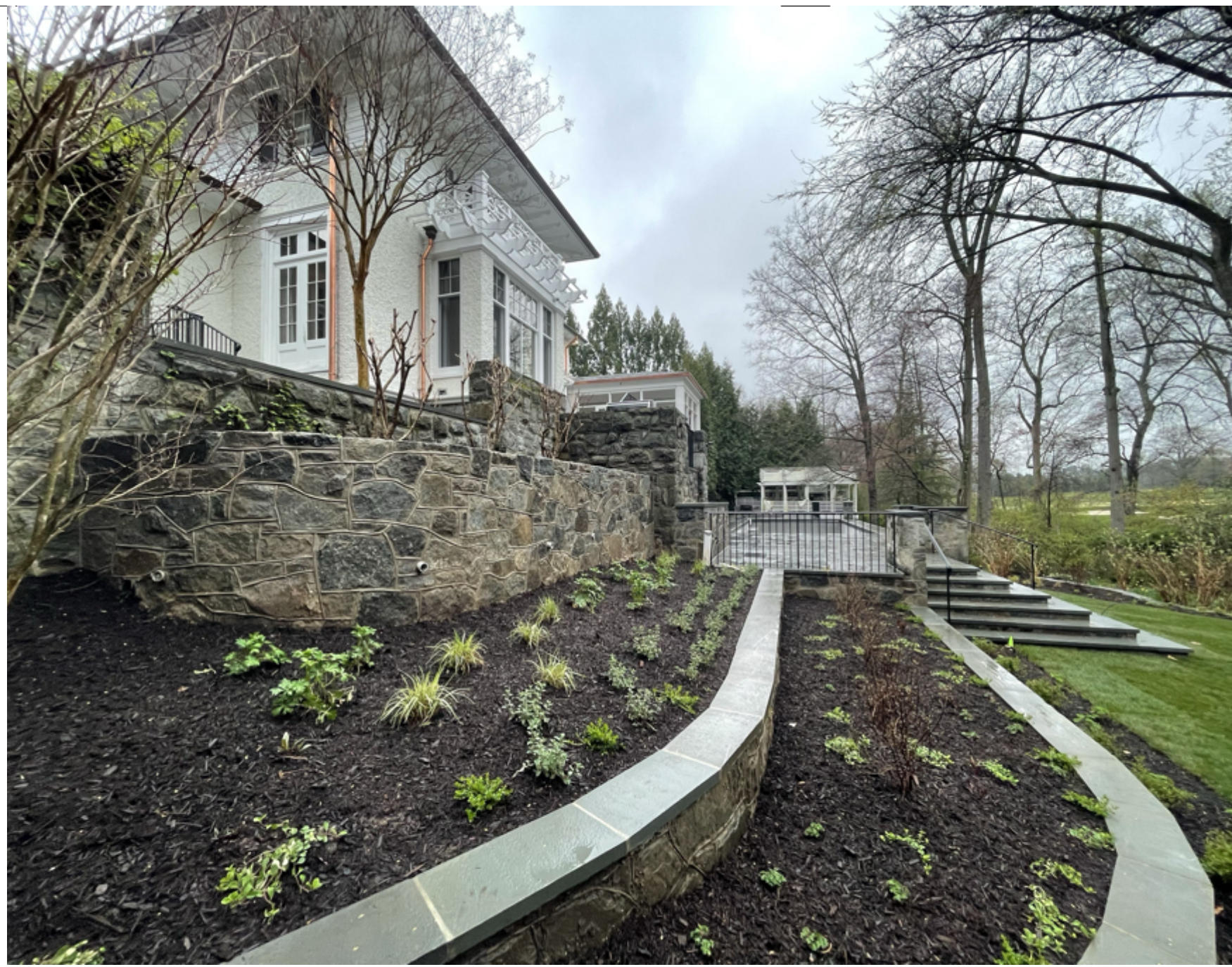
EXISTING TERRACE WALLS FROM REAR LAWN
