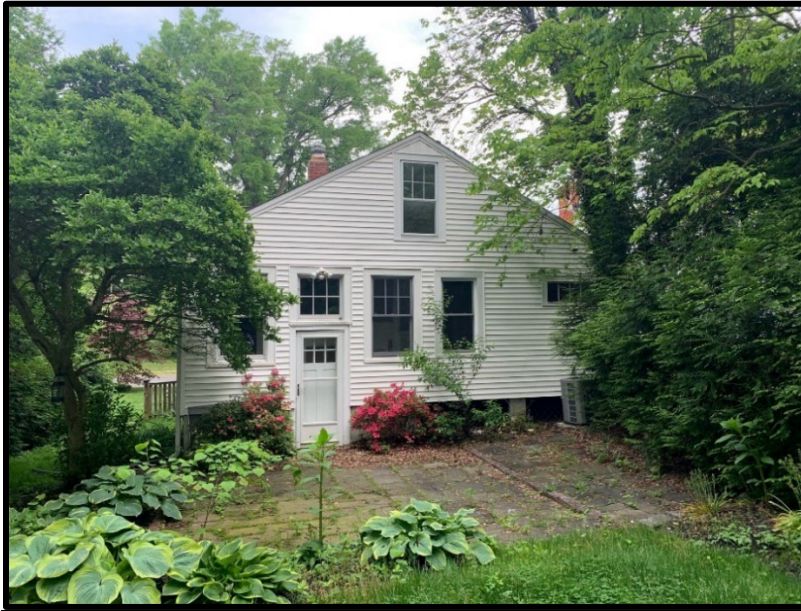
Figure 4: The rear elevation of 10305 Armory Avenue.
