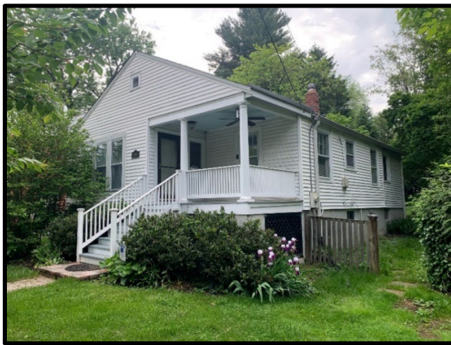
Figure 3: The front and the right-side elevations of the residence at 10305 Armory Avenue, Kensington.
