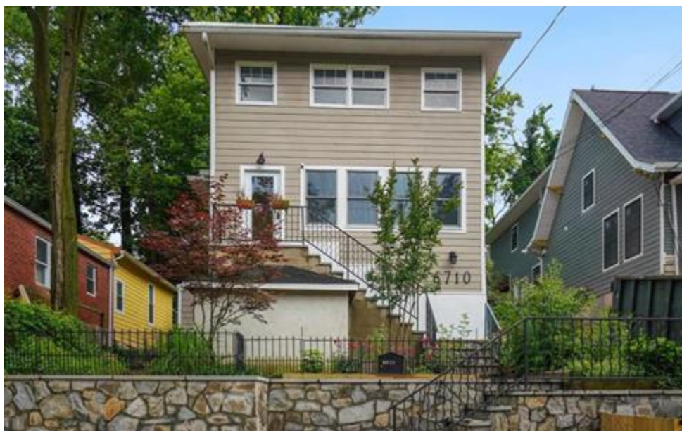
Figure 2: Existing front elevation of the subject property.
