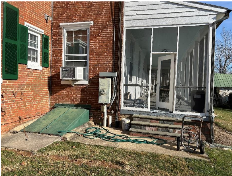
West Porch Stair
