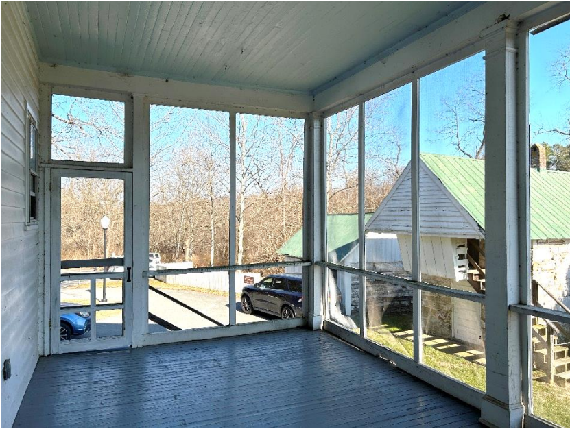
East Porch Entry, Looking towards Dairy and Parking
