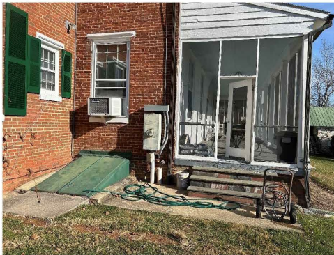
West Porch Stair
