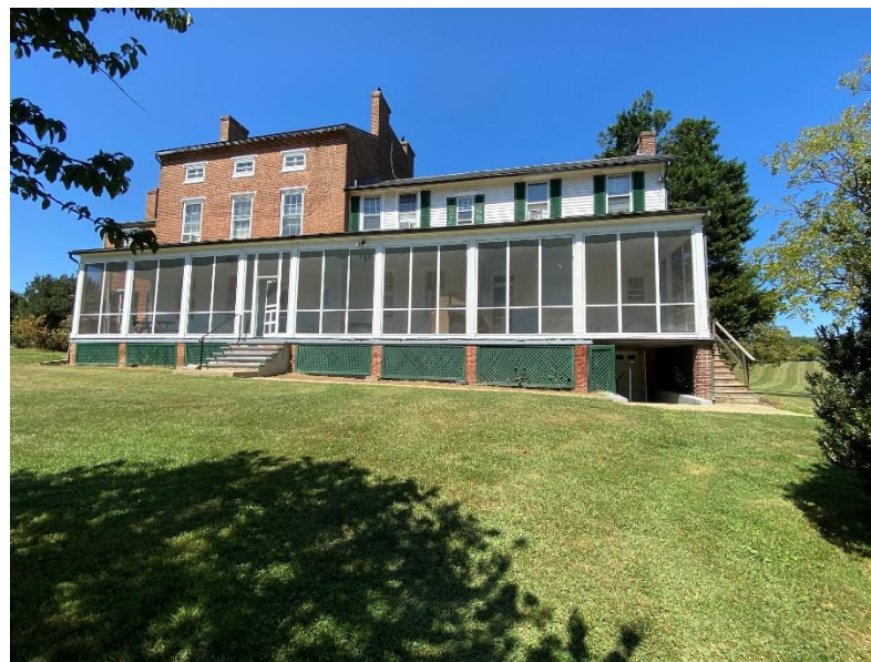
Rear (South) Elevation – Primary Entrance at Center Porch Steps
