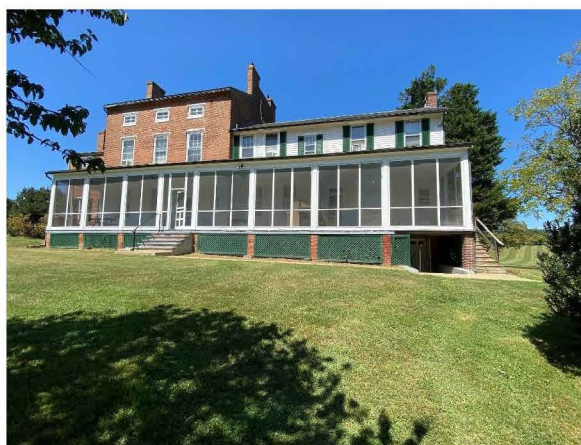
Rear (South) Elevation – Primary Entrance at Center Porch Steps
