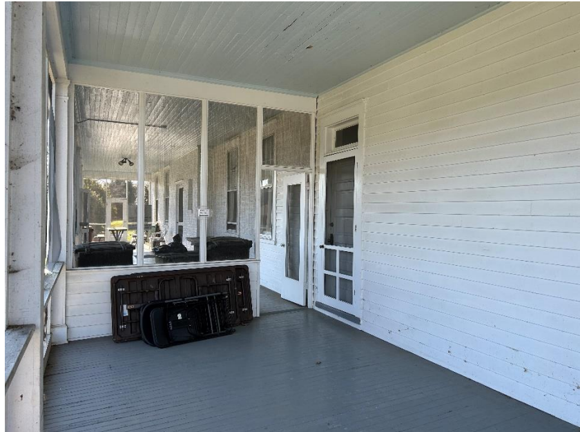
East Porch, Looking West to Kitchen Door
