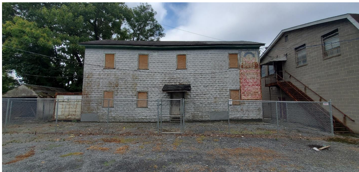
Figure 4: View of the facade of Hoyle's Mill, 2023.
