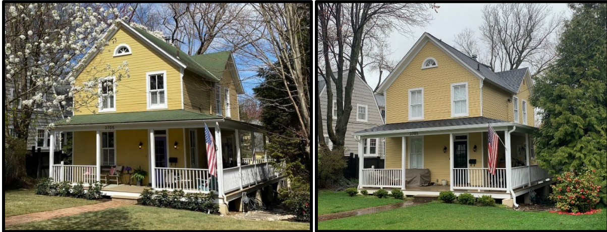
Figure 10: The real estate listing photo from 2020, left, shows the previous 3-tab shingle roof that has since been replaced with an architectural grade shingle roof as seen in the existing photo on the right. Source: Bright MLS
