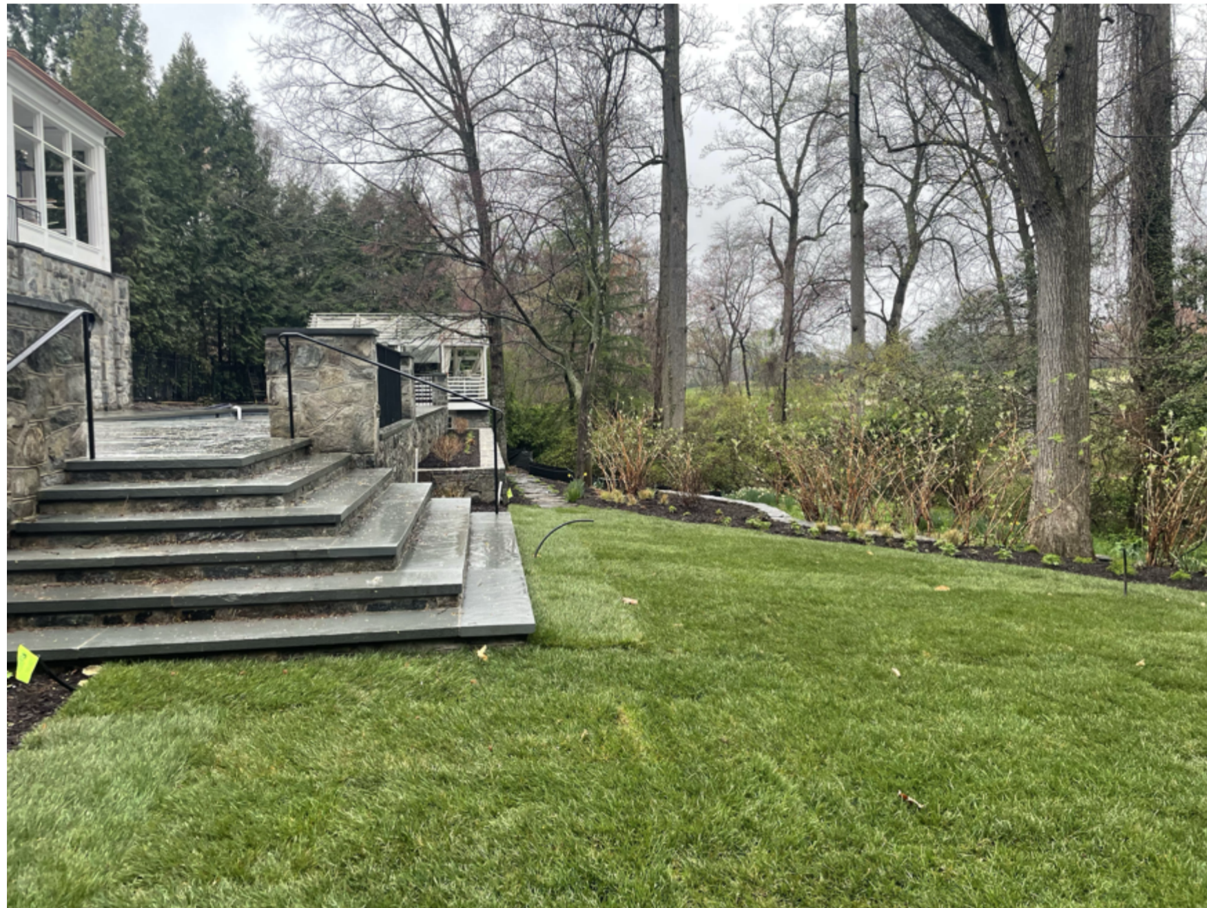
EXISTING STAIRS TO LOWER LAWN
