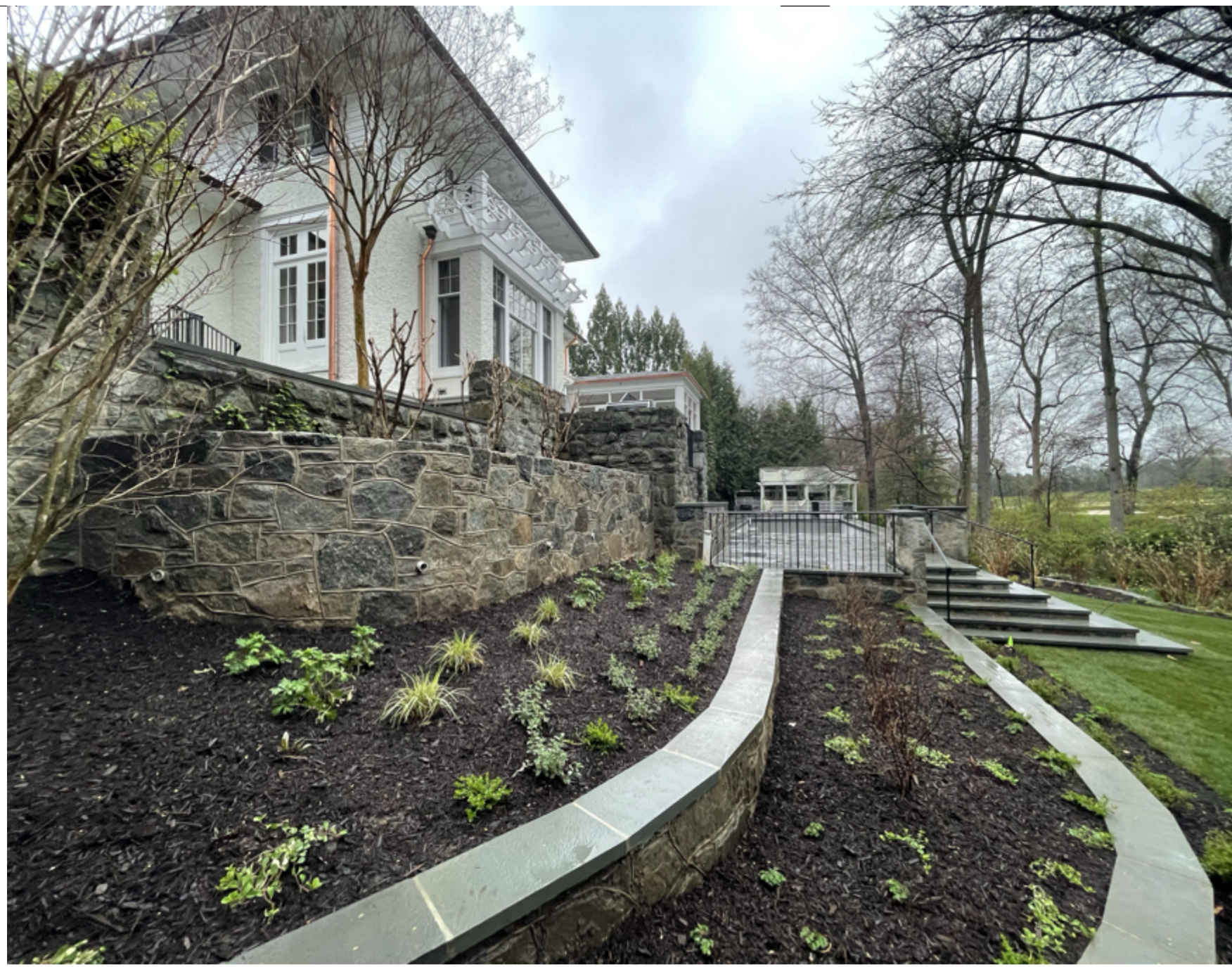
EXISTING TERRACE WALLS FROM REAR LAWN
