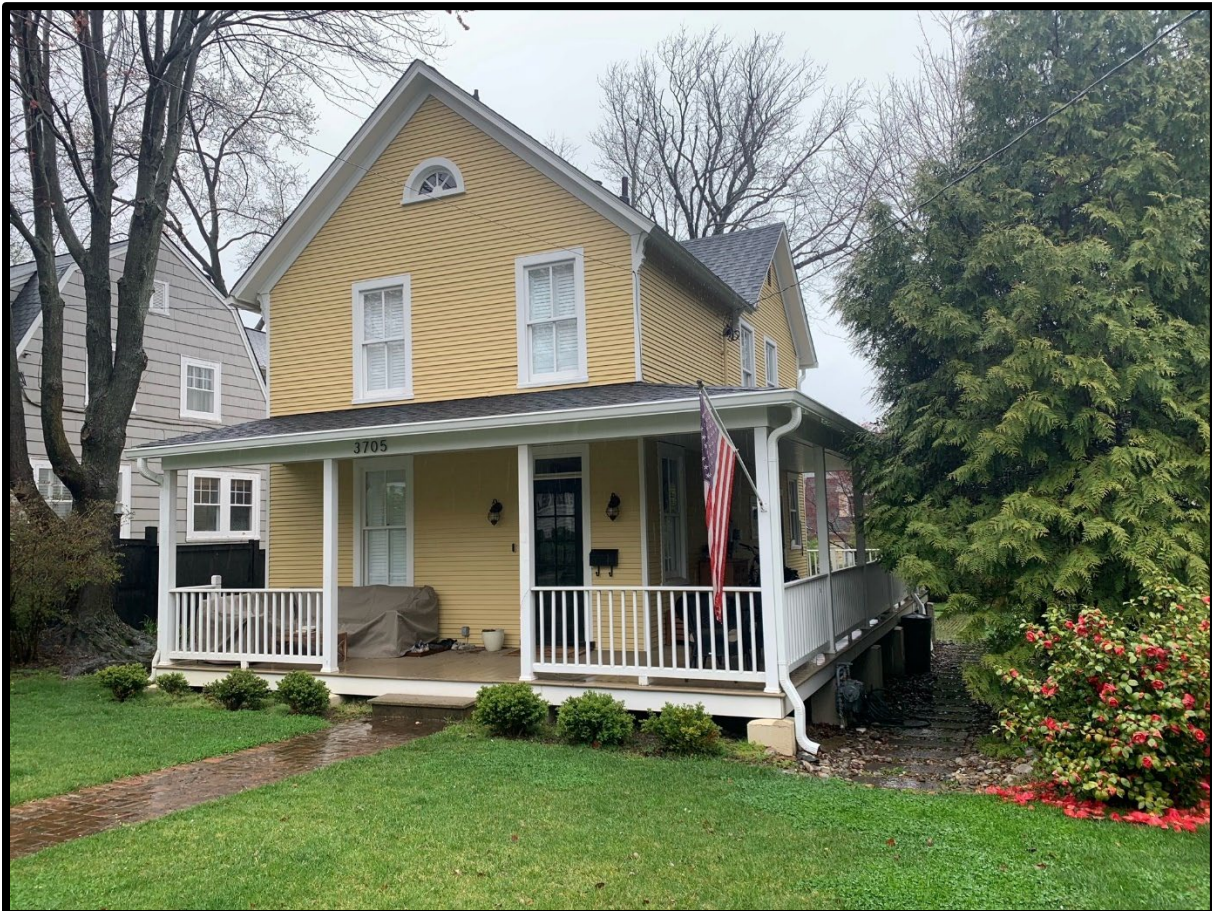
Figure 2: The front and right-side elevations of 3705 Underwood St.
