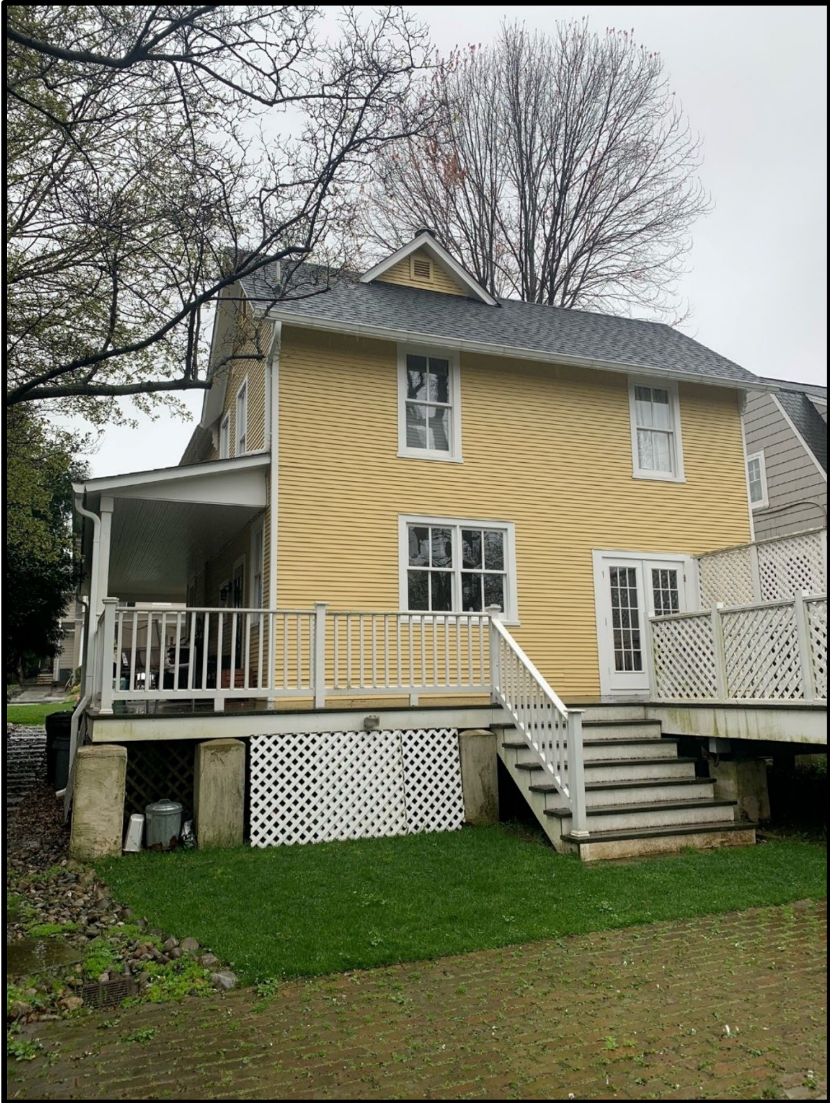
Figure 3: The rear and right-side elevations of 3705 Underwood St.
