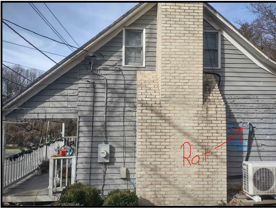
Figure 7: The applicant provided this annotated photo of the right-side elevation.
