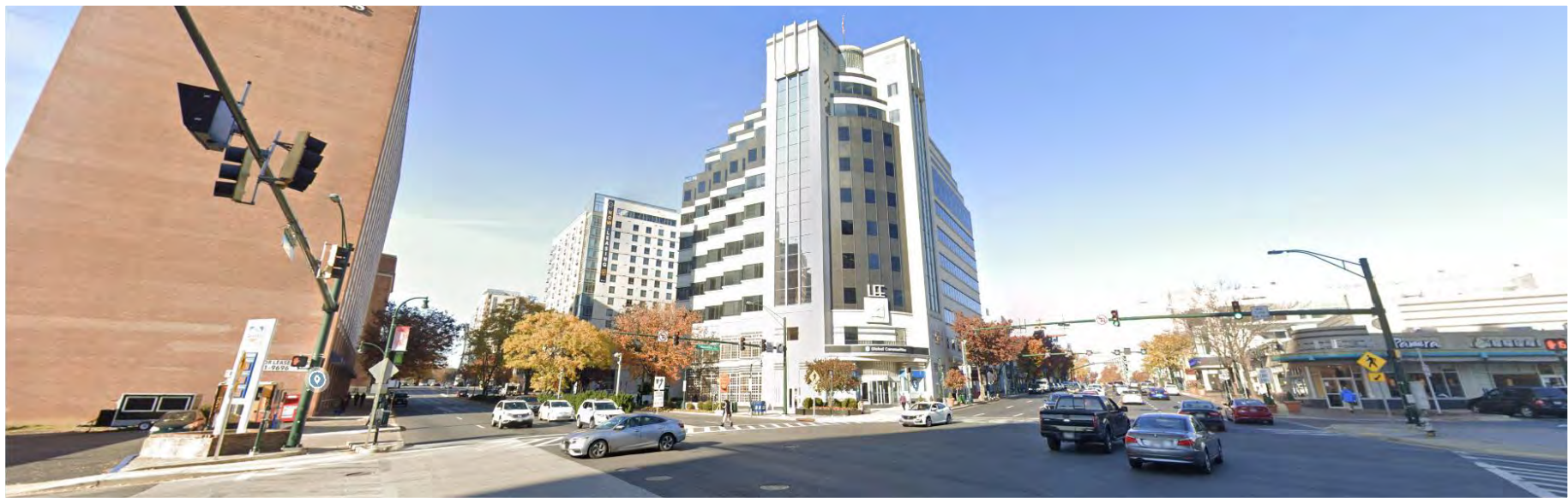
VIEW C - GEORGIA AVE / COLESVILLE ROAD VIEW
