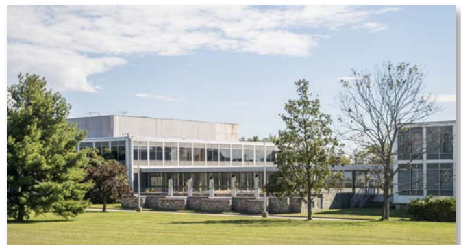
Verizon's Fairland Data Center
