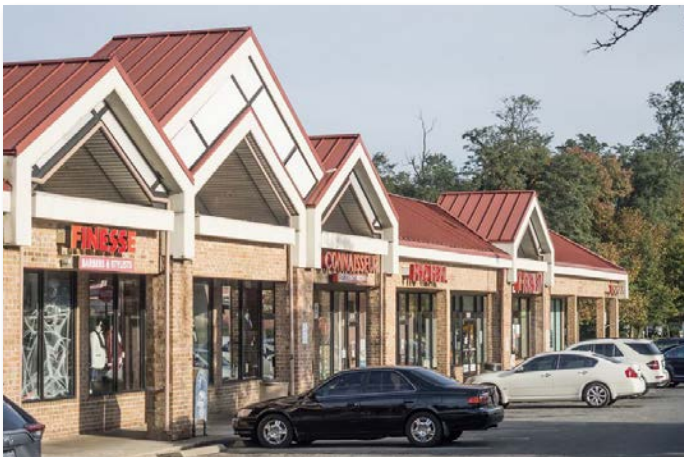
Storefronts of the Briggs Chaney Center with parked cars
