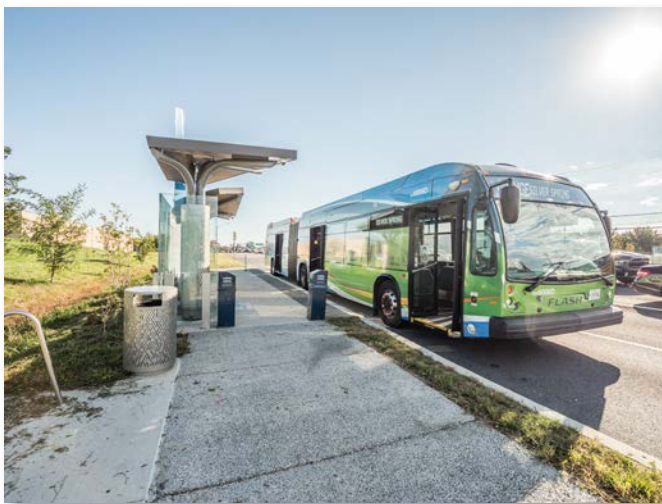
Flash BRT bus at a station on U.S. 29 (Columbia Pike)
