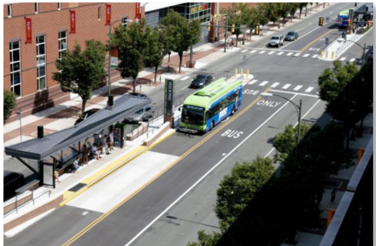
Median Bus Rapid Transit station in Richmond, VA
