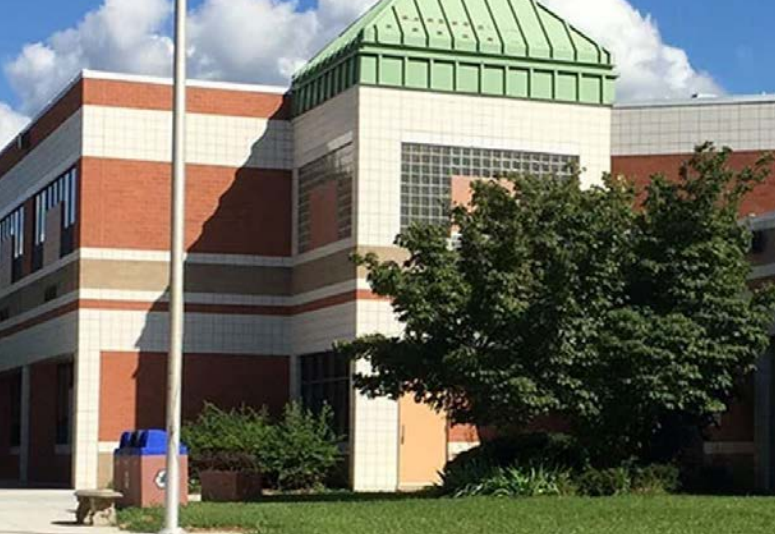
Greencastle Elementary School
