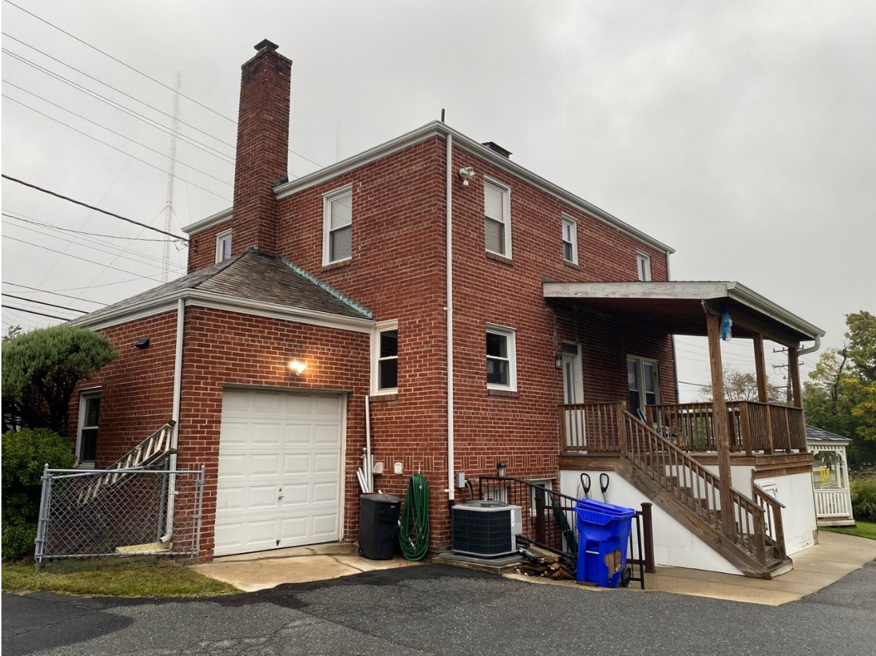
Figure 3: View of the south (rear) and west elevations of the Romeo and Elsie Horad House looking northeast from the driveway, 2023. Source: Ottery Group.
