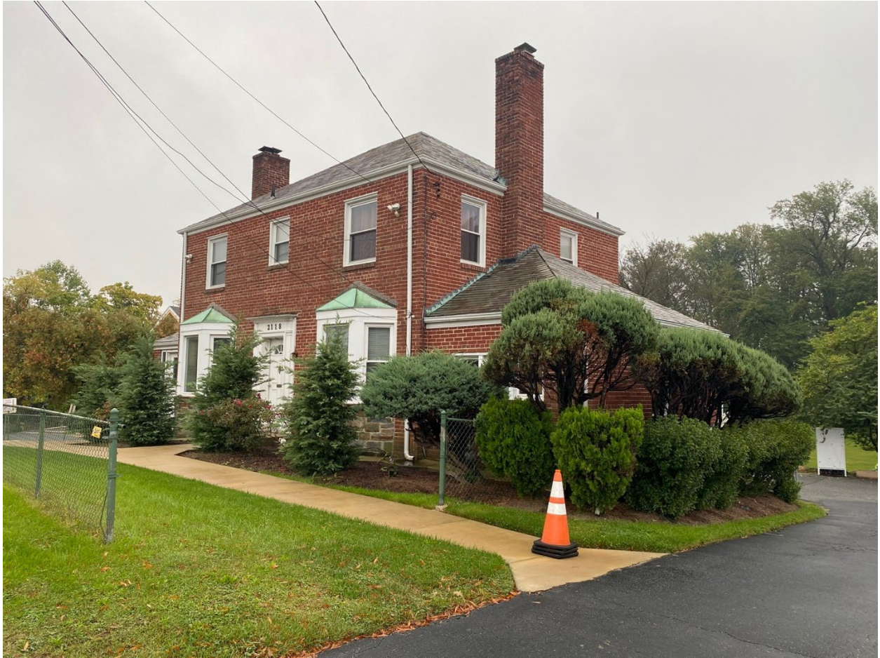
Figure 2: View of the north (façade) and west elevations of the Romeo and Elsie Horad House looking southeast from the sidewalk of University Boulevard West, 2023. Source: Ottery Group.
