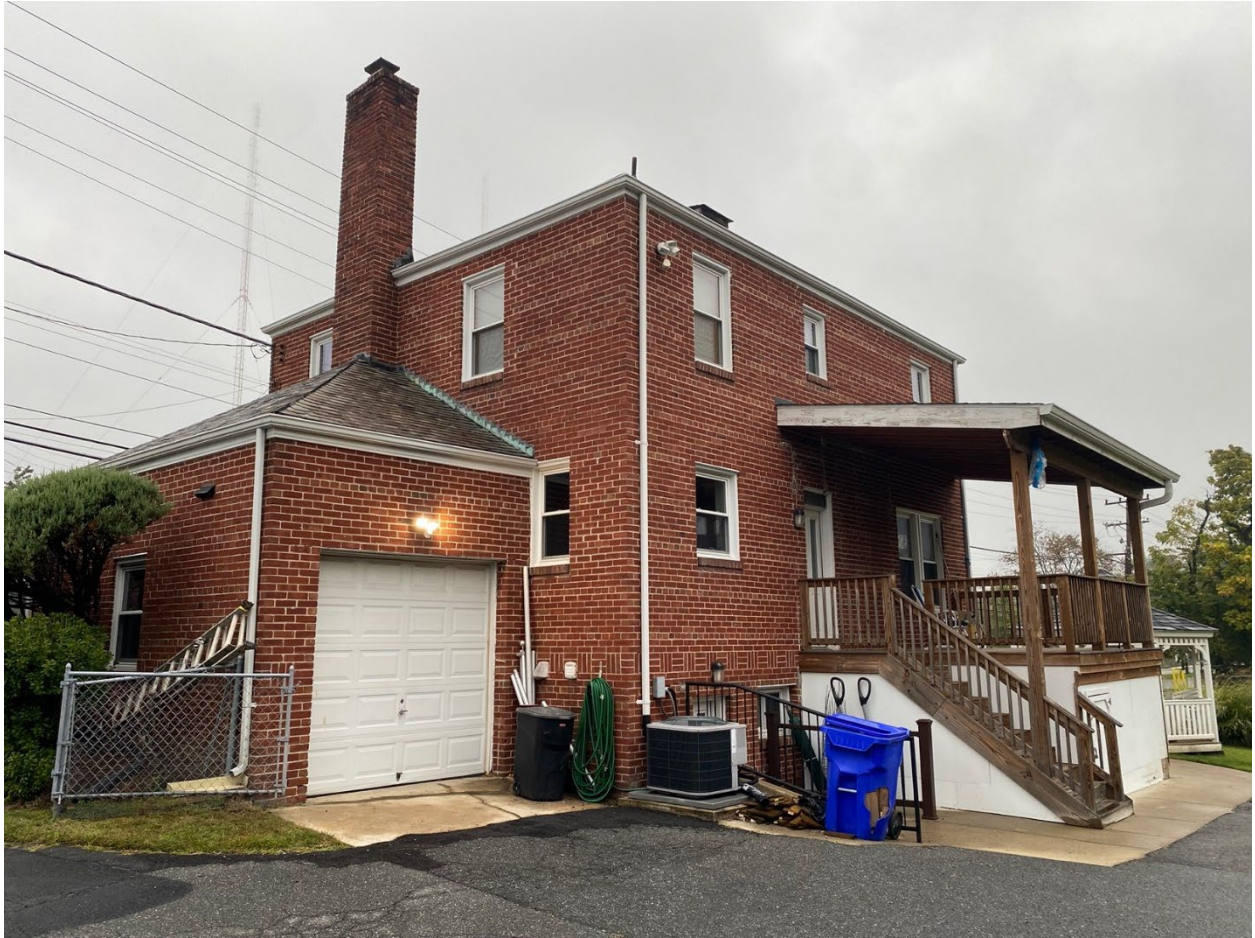
Figure 3: View of the south (rear) and west elevations of the Romeo and Elsie Horad House looking northeast from the driveway, 2023. Source: Ottery Group.
