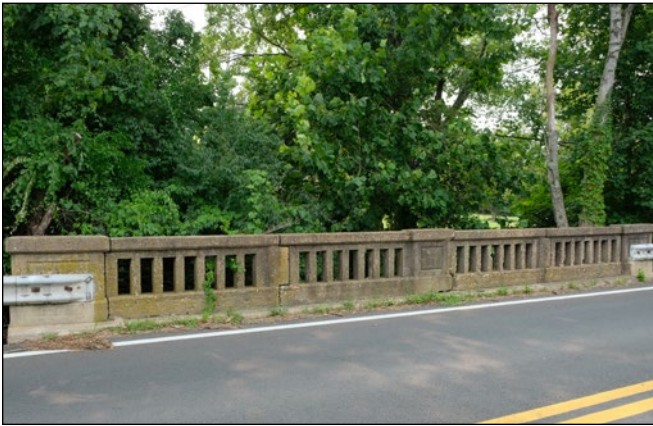
Bucklodge Road Bridge
