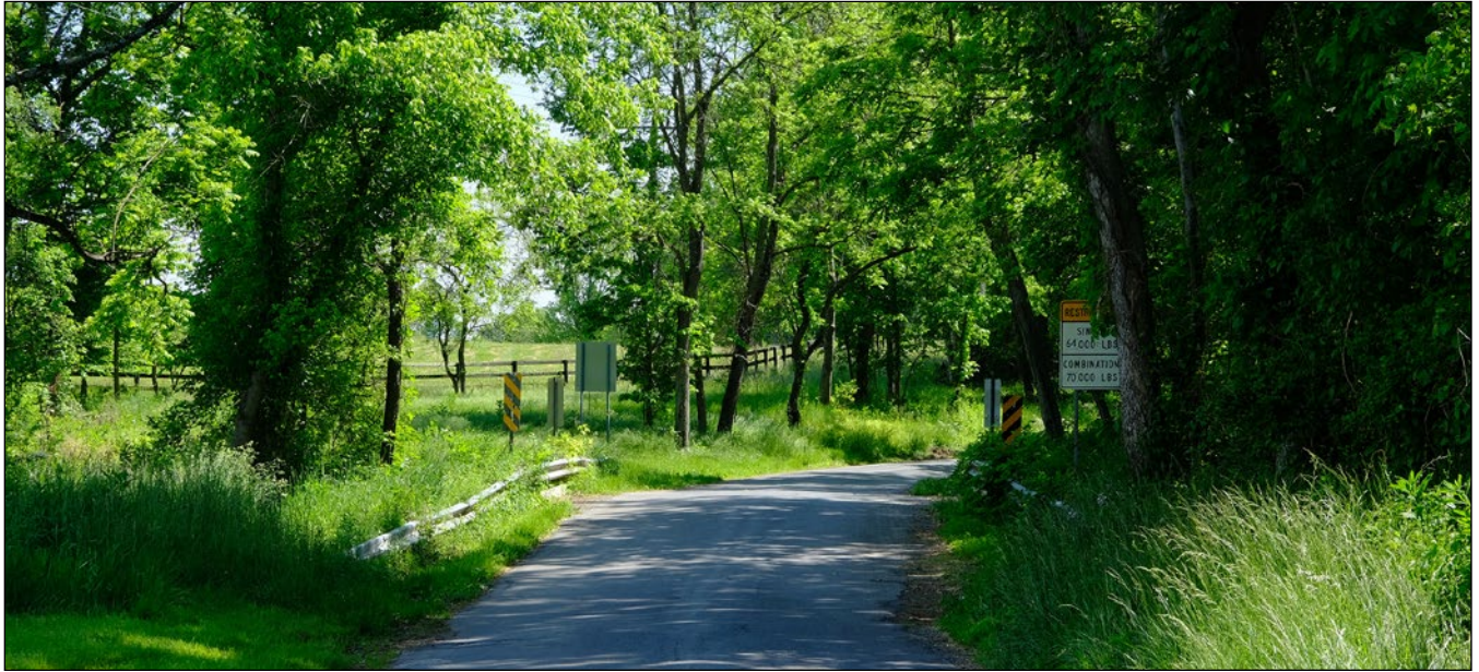
Narrow bridge along Edwards Ferry Road
