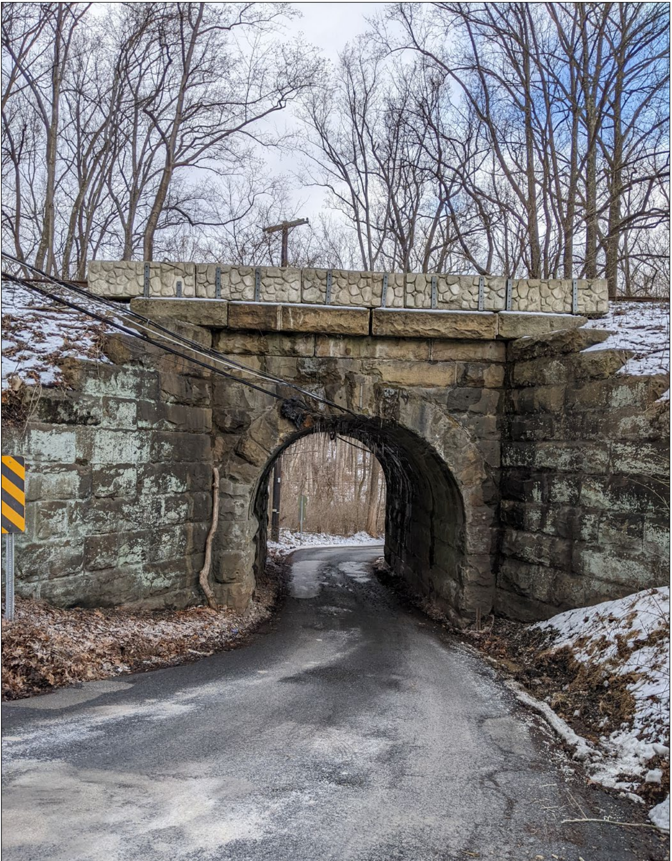
CSX Underpass on Game Preserve Road
