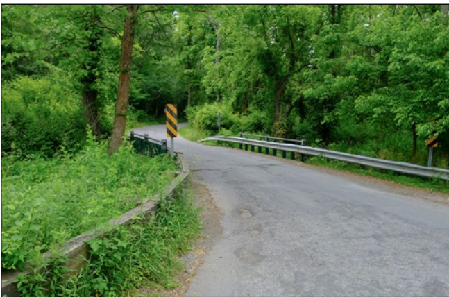
Narrow bridge on Howard Chapel Road crossing over the Hights Branch
