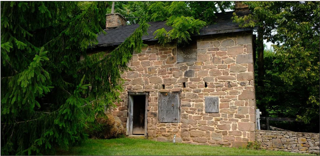
Seneca sandstone building close to road that is believed to have housed enslaved people at the Richard T. White house
