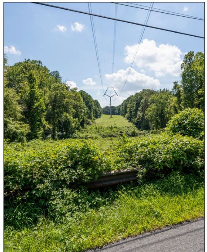
View of power line opening along Tucker Lane
