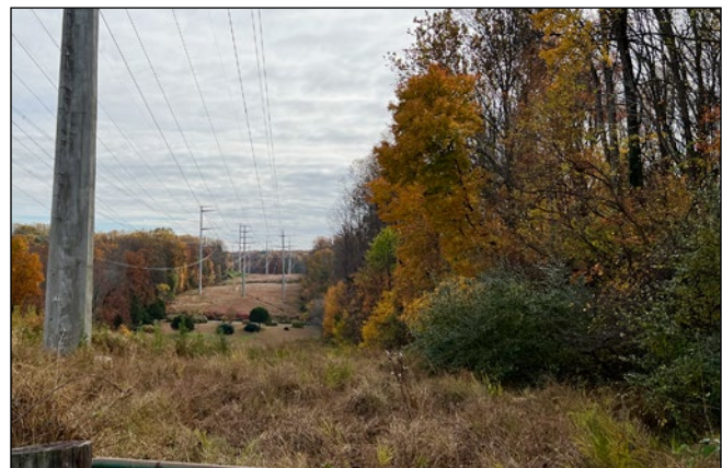
Distant view along the power lines
