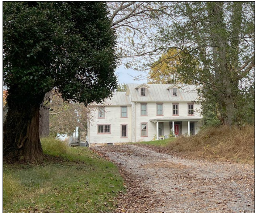
Built in 1882, Oakleigh is a historic five bay, Victorian house.
