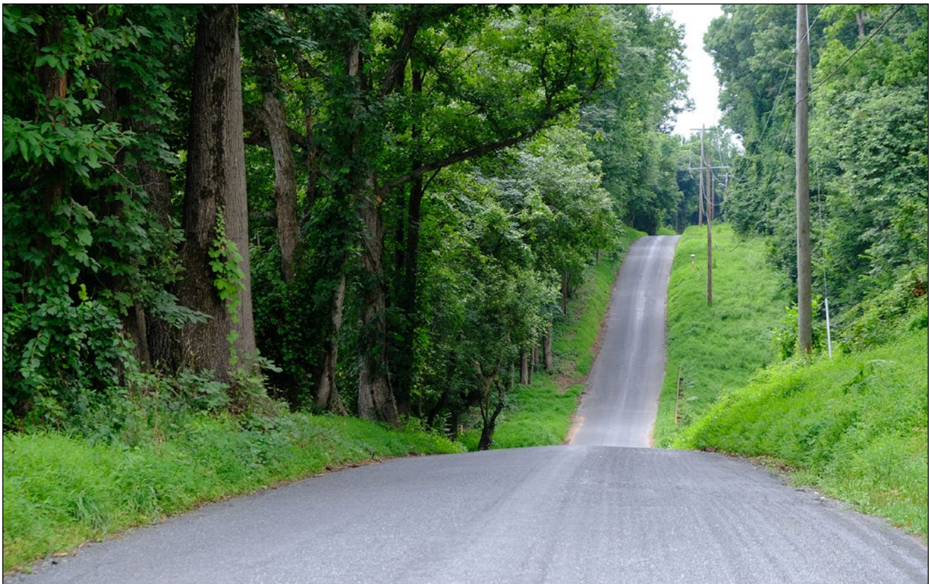
Roller coaster alignment and steep embankments along the edge of the road
