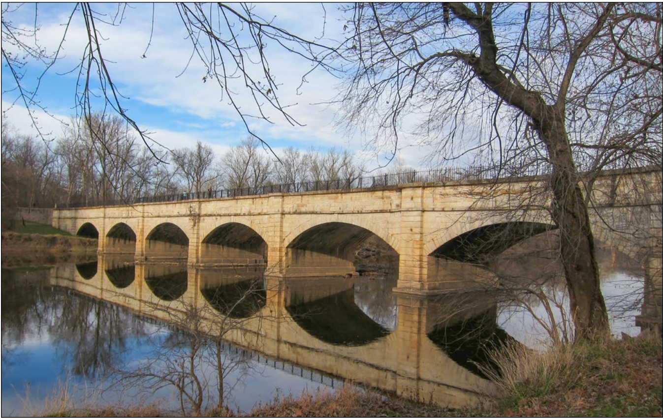
The Monocacy Aqueduct once carried the waters of the C&O Canal over the Monocacy River.
