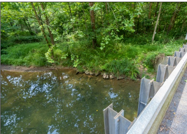
View into Scott Branch from the road
