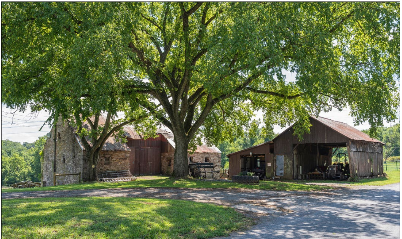
The c. 1830 stone bank barn is located on the east side of Martinsburg Road just north of the power lines.
