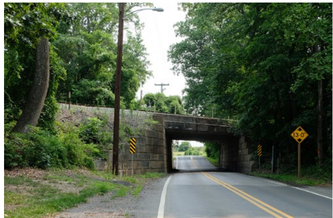
Bucklodge Road passing under the C&O railroad tracks
