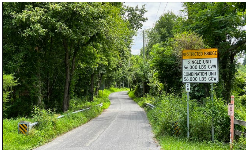
Narrow bridge leading to Seneca Creek
