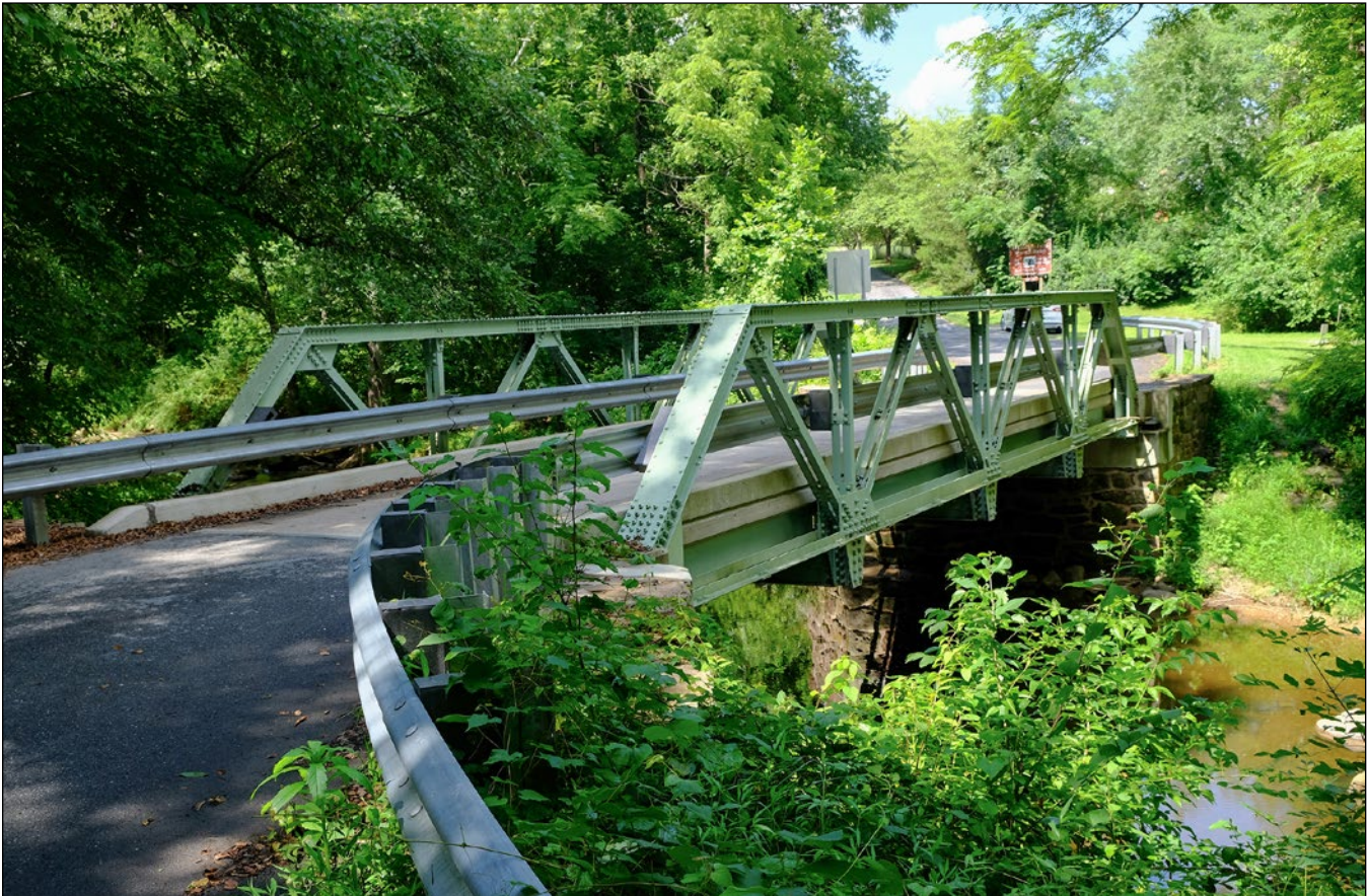
Single-lane iron truss bridge over Dry Seneca Creek
