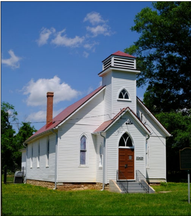
The 1903 Warren Methodist Episcopal Church in Martinsburg
