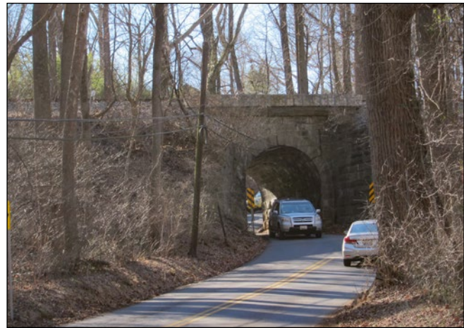
One-lane railroad underpass under Game Preserve Road
