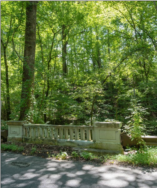
1930 concrete-panel designed bridge
