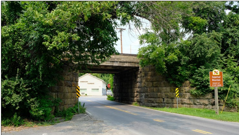
Railroad bridge within Dickerson Historic District
