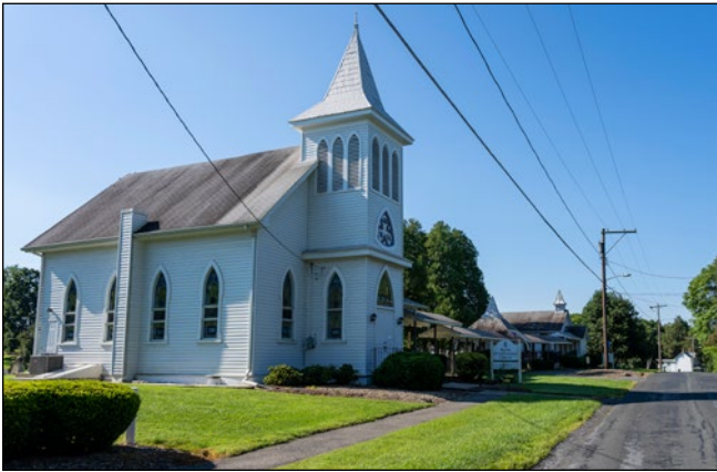
Looking south on White Ground Road toward the Boyds Presbyterian Church
