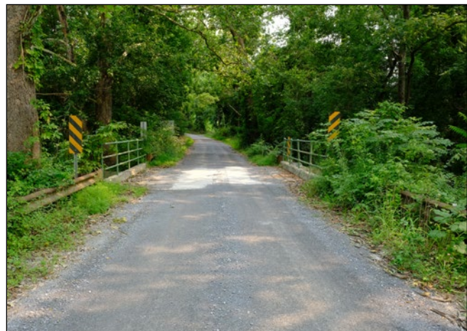
1925 metal pipe rail bridge
