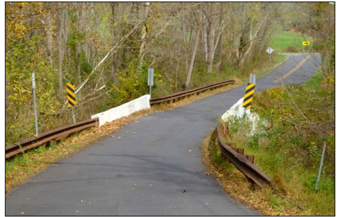
One-lane bridge on Haviland Mill Road
