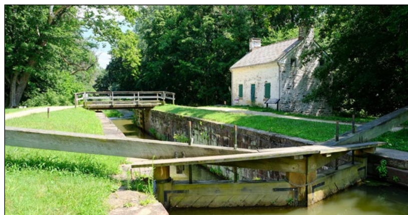
Pennyfield Lock House & Lock #22
