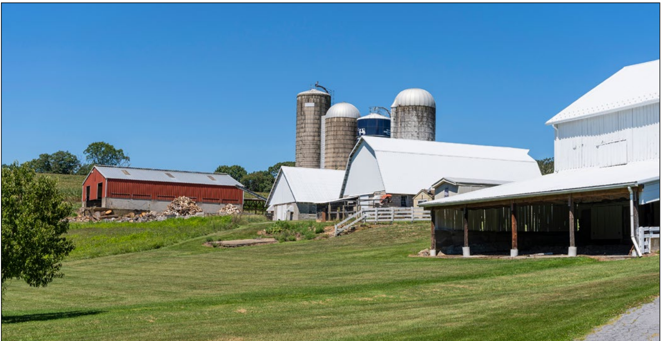
Looking east toward Kingstead Farm
