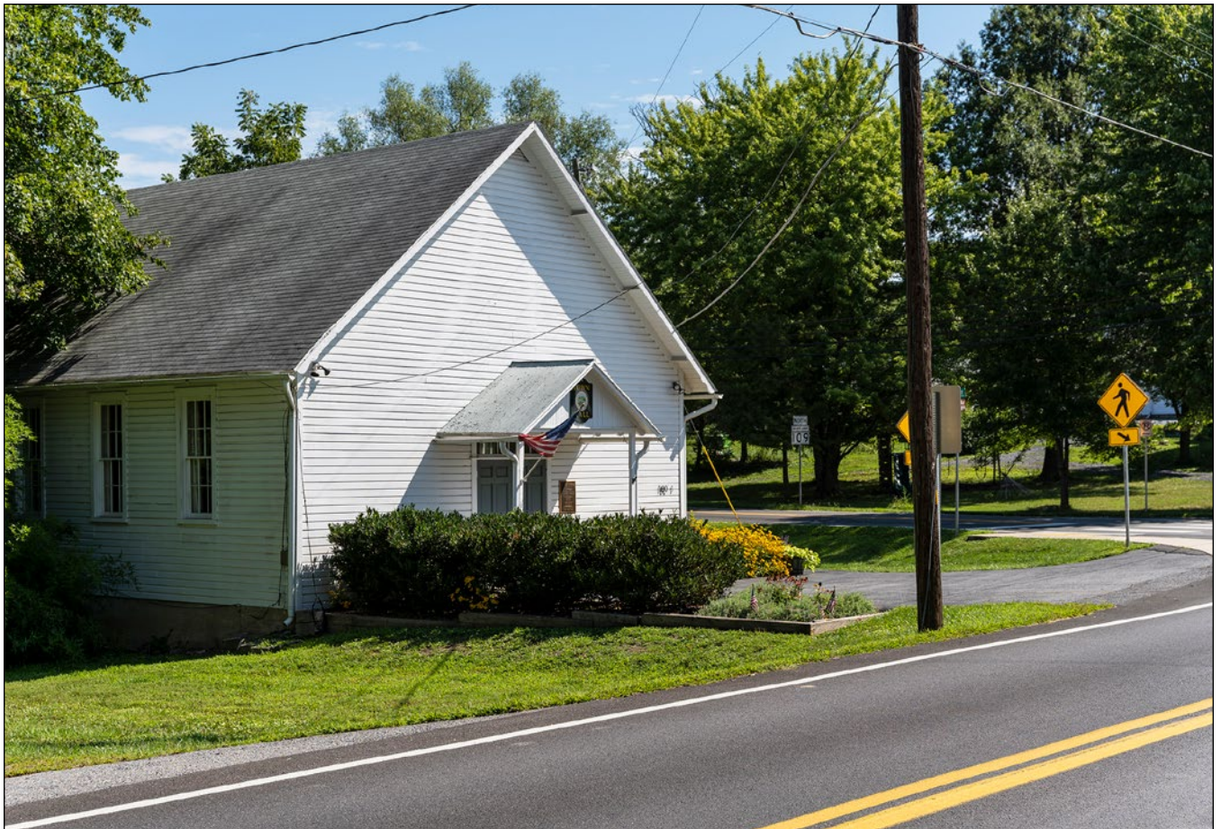
Barnesville Town Hall on the northwest corner of the intersection of Barnesville and Old Hundred Roads
