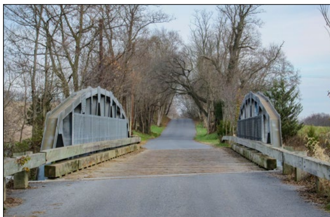
Mouth of Monocacy Road crossing over the CSX tracks
