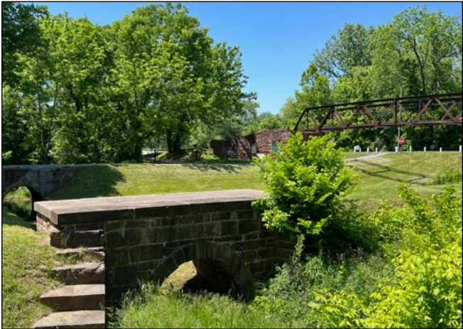
Sandstone culvert and iron bridge over the C&O Canal
