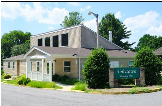
The Tobytown community located at the beginning of Pennyfield Lock Road
