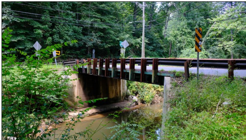
One-lane bridge over the Watts Branch
