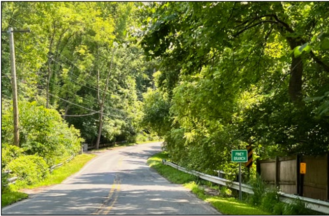
Looking south on the exceptional rustic section of Glen Mill Road just north of the Piney Branch
