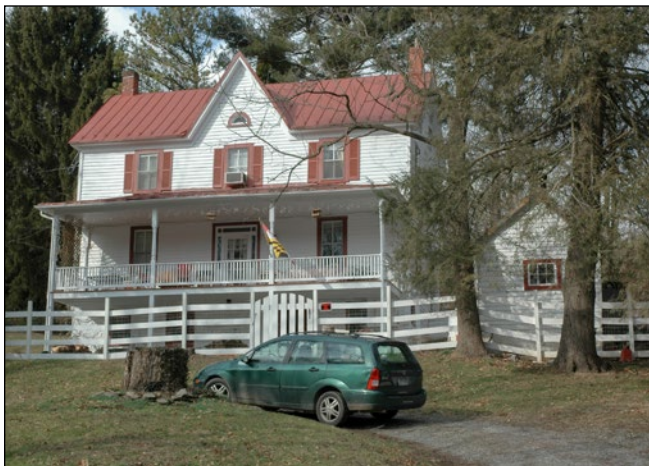
Believed to have been built around 1903, the Chrobot House is constructed in a Germanic tradition with an exposed stone foundation on the front facade and two entry doors at the basement level.
