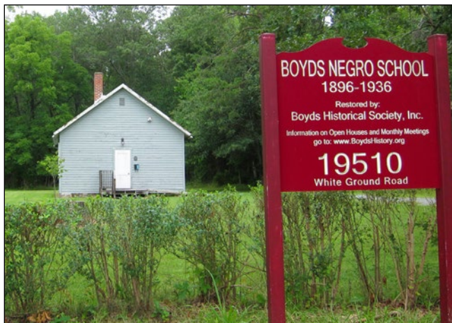
The Boyds Negro School located in the southern portion of the Boyds Historic District
