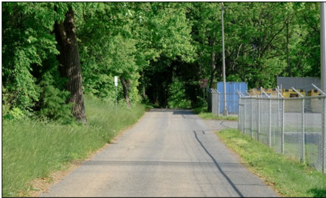
Beginning of Jonesville Road adjacent to Montgomery County depot facility
