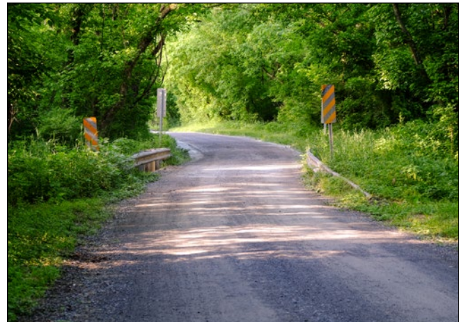
The northern one-lane bridge along the road
