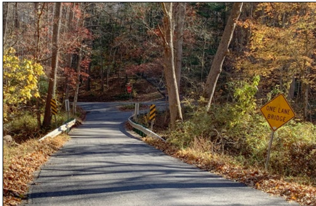
One-lane bridge over Wildcat Branch
