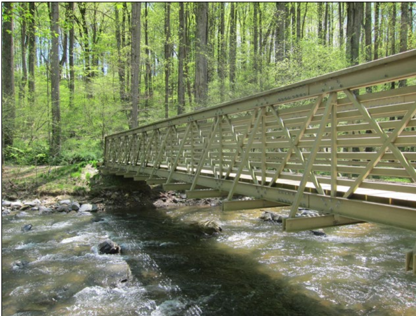
Pedestrian bridge over Little Bennett Creek
