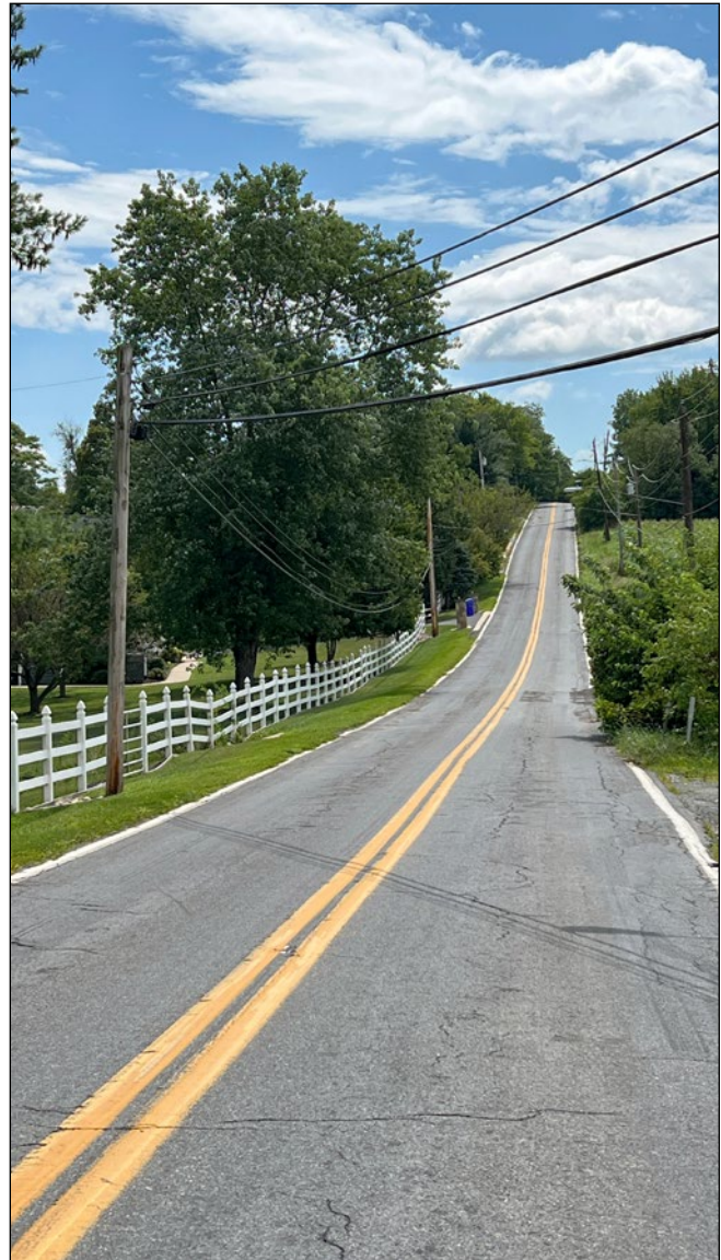
Looking south on Prices Distillery Road just south of the intersection with Clarksburg Road
