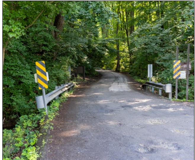
One-lane bridge leading to the C&O Canal parking lot
