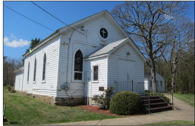
St. Mark's United Methodist Church located on the west side of the road in the Boyds Historic District
