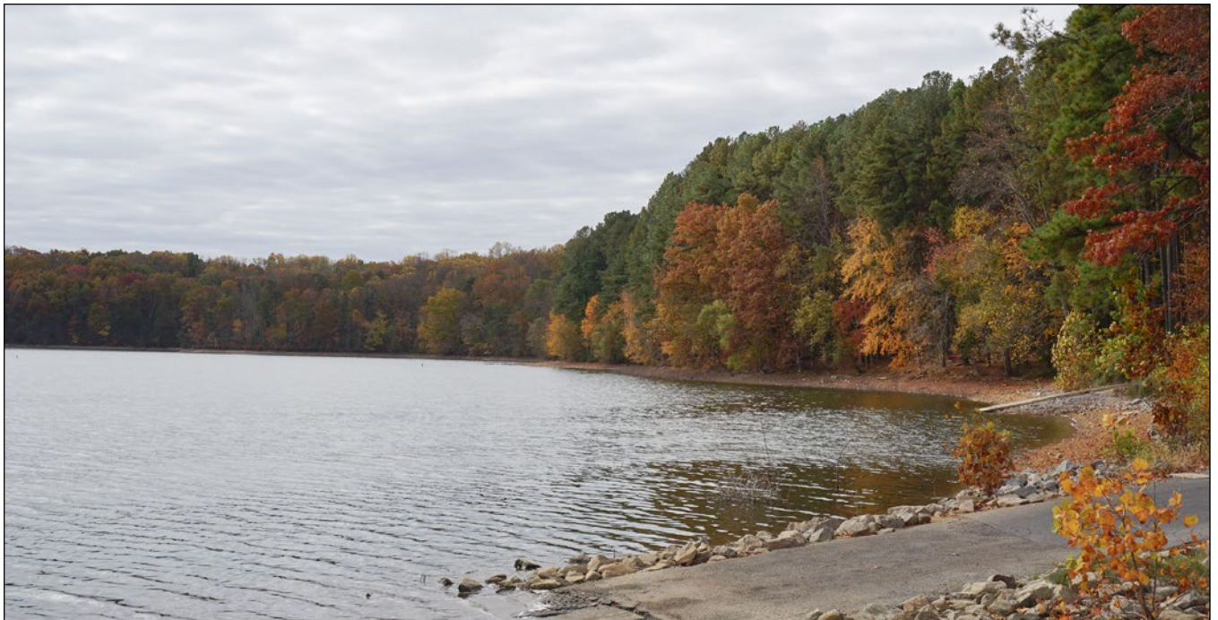
Boat ramp on the Triadelphia Reservoir
