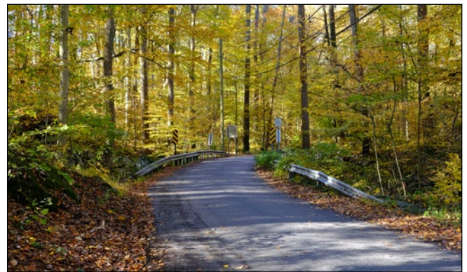
Narrow bridge crossing the Gregg Road Tributary
