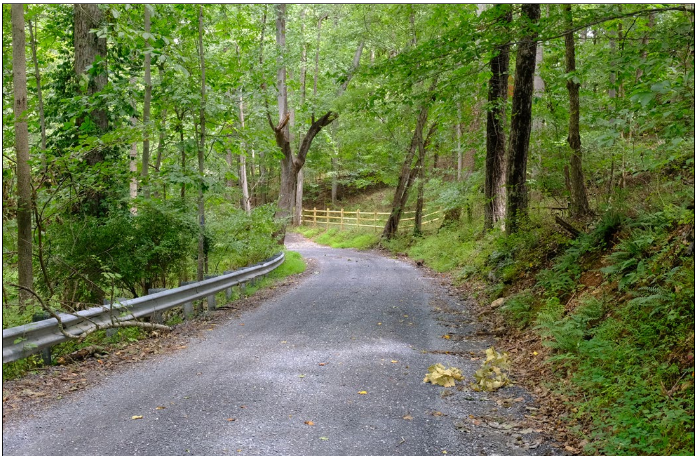
Gravel portion of Haines Road near the County line
