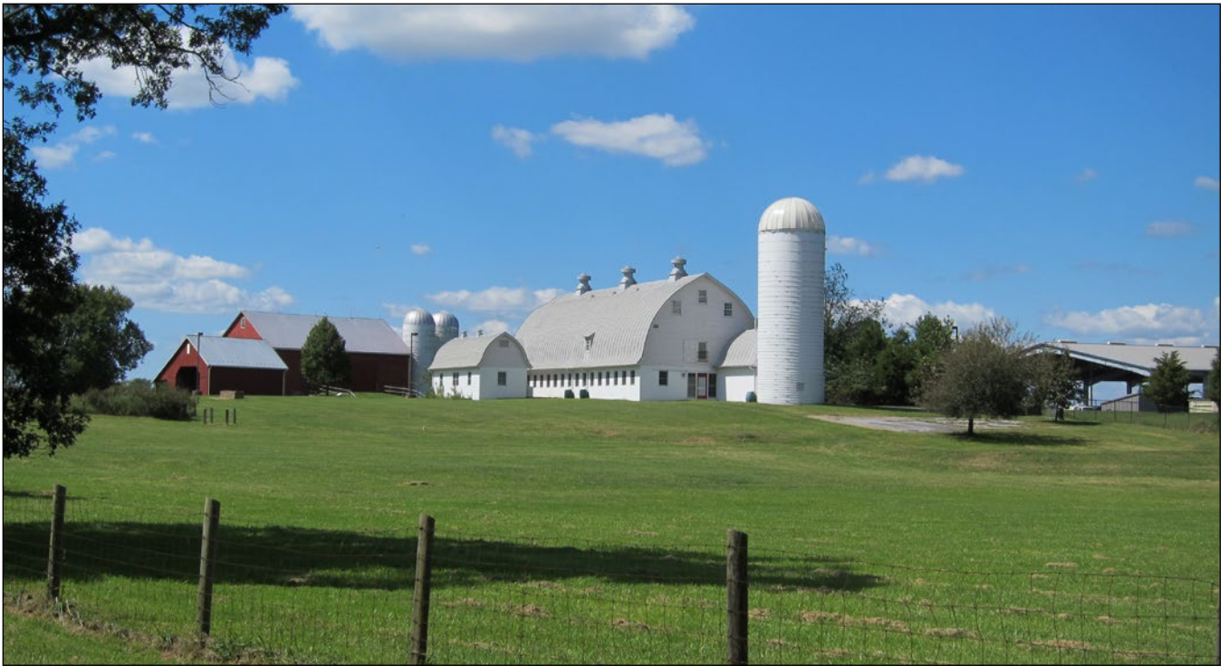
The Lawrence White Barn located on the northern end of Martinsburg Road
