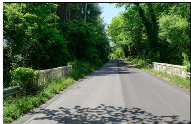
The 1931 concrete-paneled bridge just west of Wasche Road
