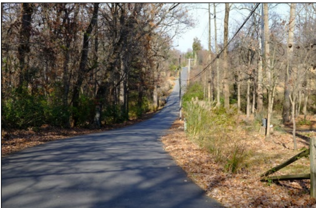
Rolling alignment of Santini Road
