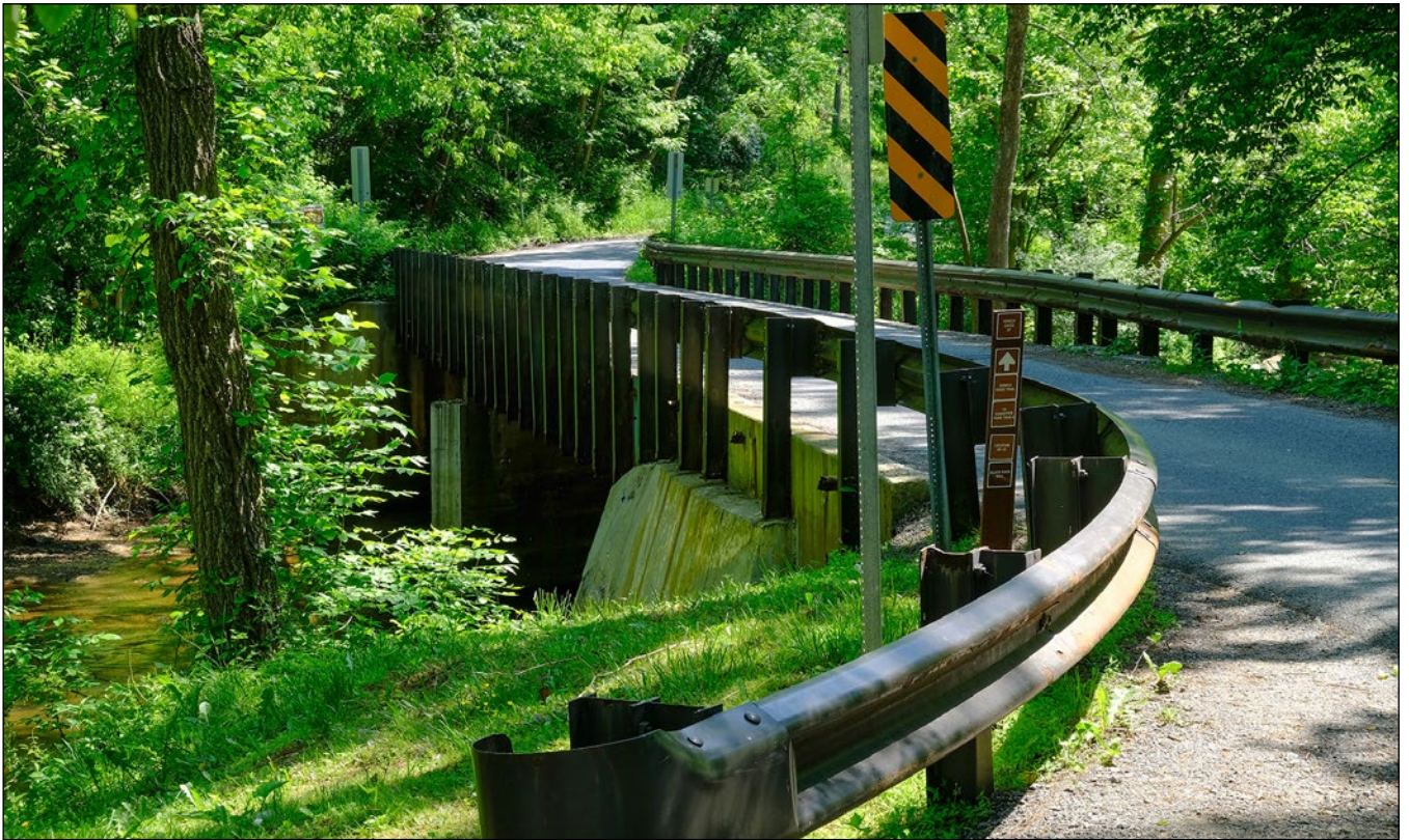
One-lane steel bridge crossing Great Seneca Creek
