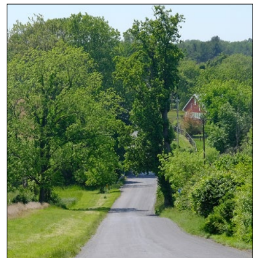
Sloping of Club Hollow Road traveling west
