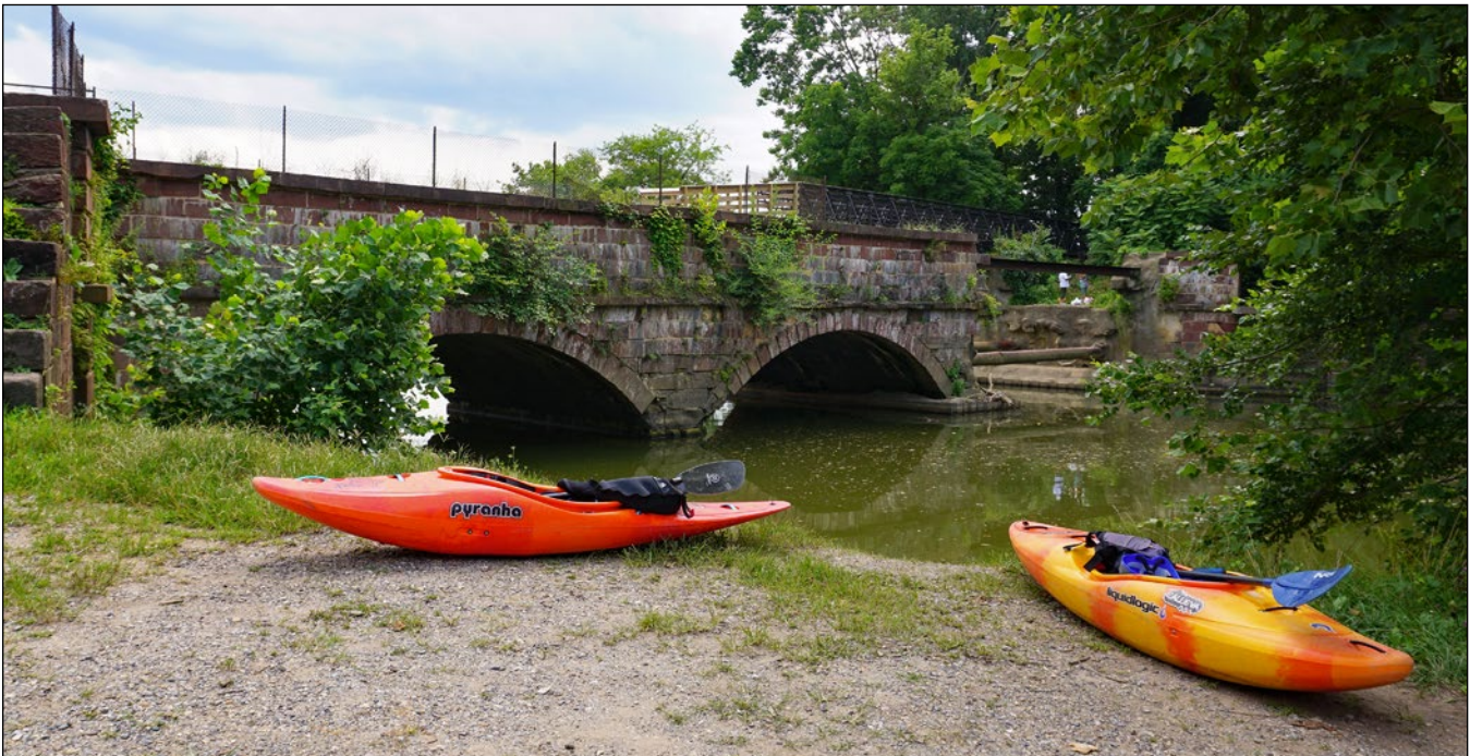
Seneca Creek Aqueduct
