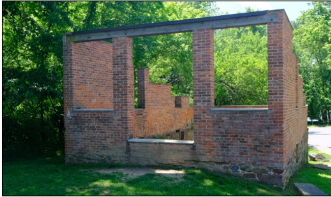
Ruins of the 1850 Edwards Ferry Brick Store
