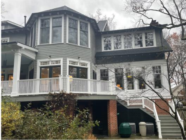
Figure 3: A small section of the deck and the stairs will be demolished.
