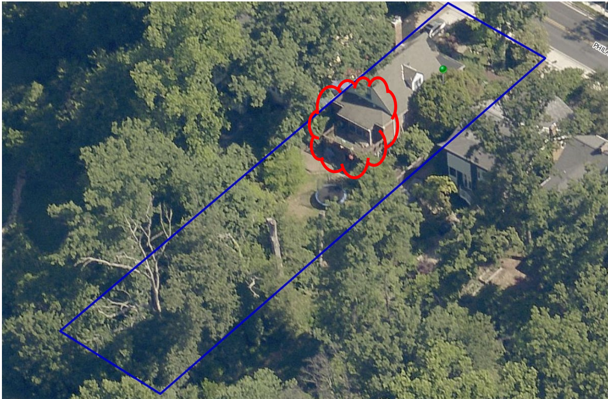
Figure 6: The subject property is outlined in blue. The deck and one-story rear addition to be demolished are clouded in red. Source: CONNECTExplorer.
