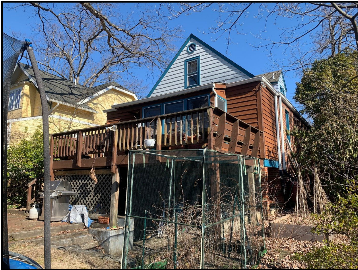
Figure 4: The rear elevation includes the addition, which is covered with wood siding, and a deck.
