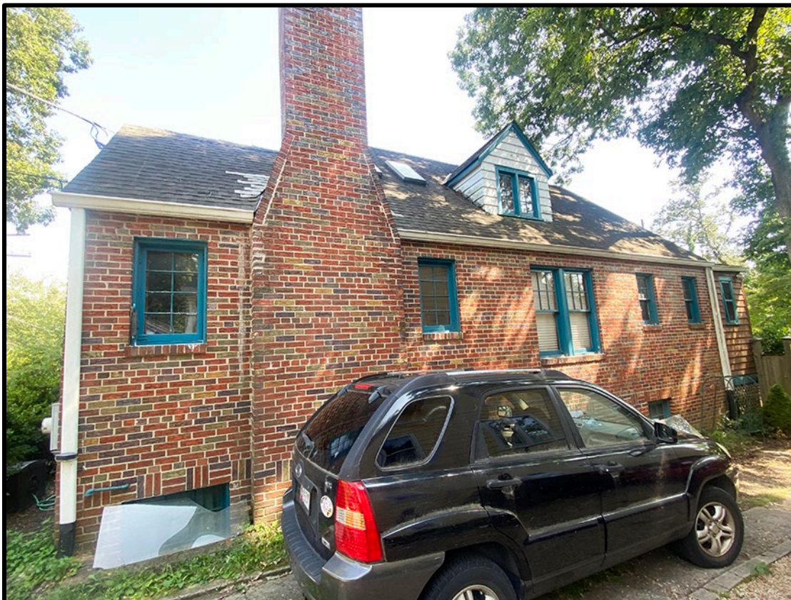
Figure 3: The right-side elevation along the driveway.
