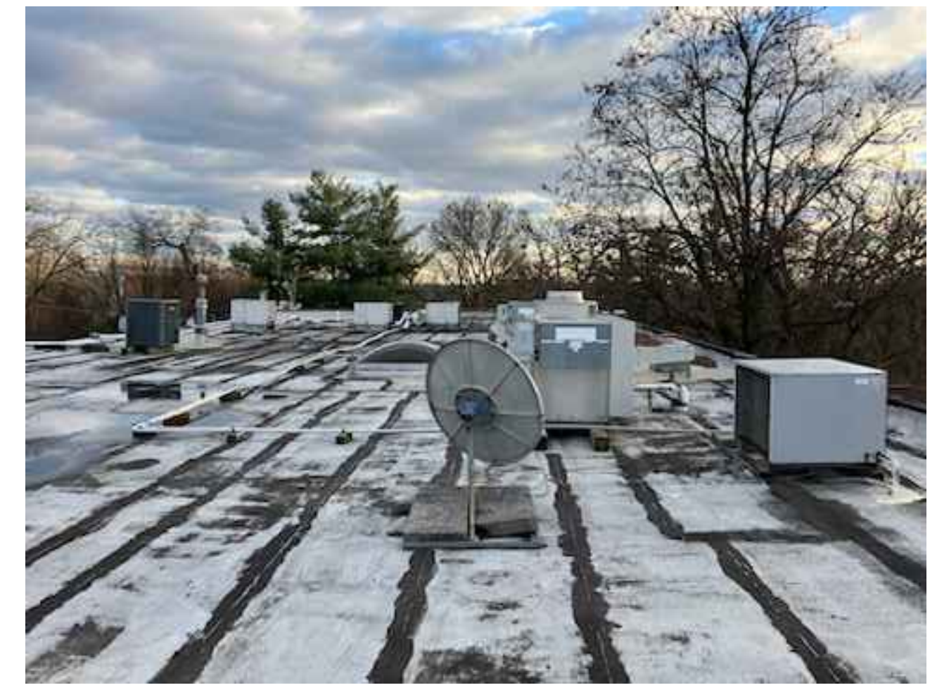
ALL ROOF EQUIPMENT SHOWN IN PHOTO TO BE REMOVED.
