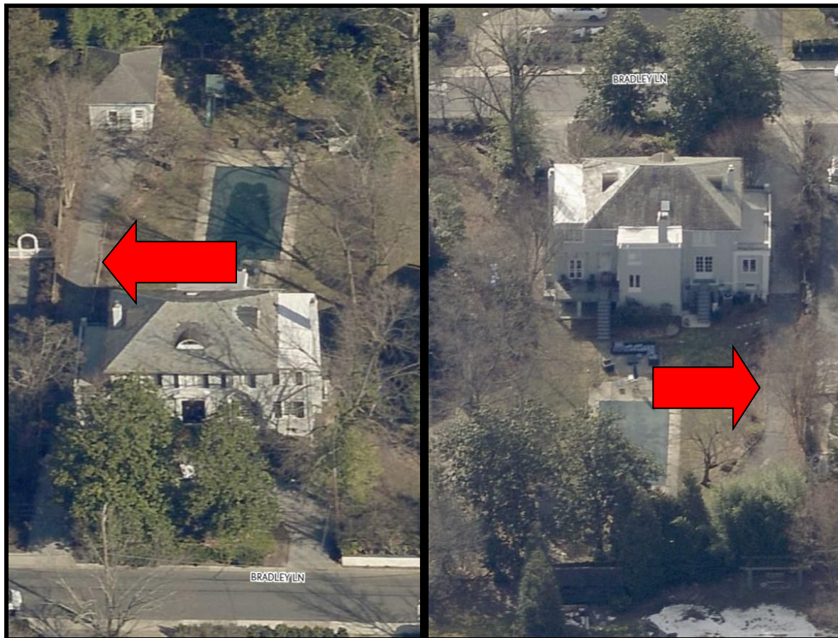
Figure 2: The driveway is indicated with a red arrow in these aerials from the front, left, and rear. Source: CONNECTExplorer
