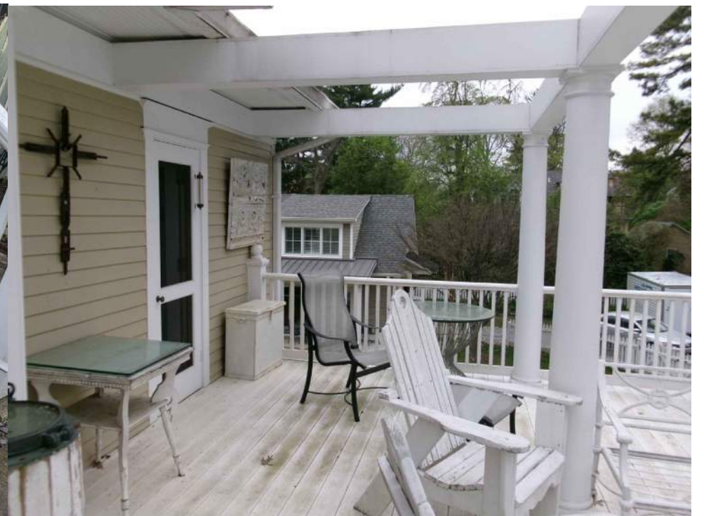
SECOND FLOOR ROOF DECK WEATHERING
