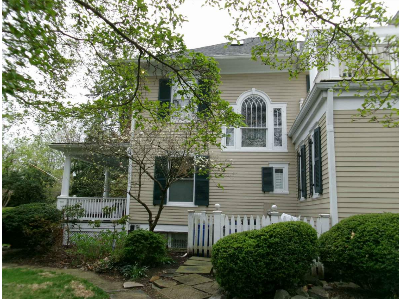
EXISTING CONDITIONS PHOTOS - TRASH AND MECHANICAL ENCLOSURE
