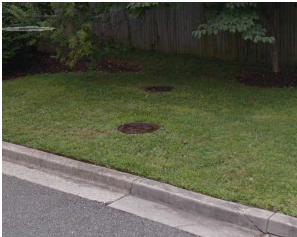
Photo 2: Example of a manhole in grass.
