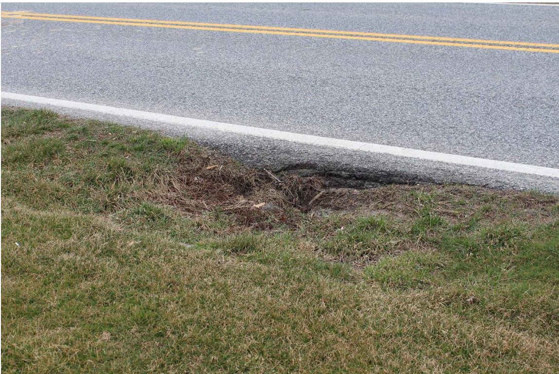
Photo 4: Existing culvert at north end of Woodlawn property (RK&K, March 2021)
