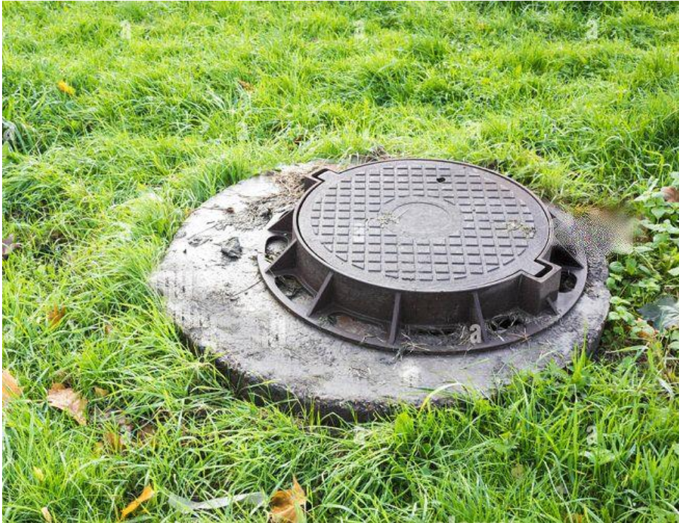
Photo 3: Example manhole cover.
