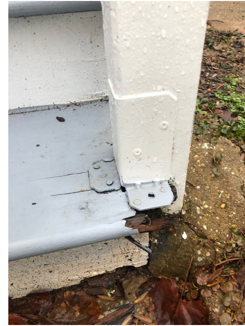
Rotted and damaged right banister, seen at its base on lower step.
