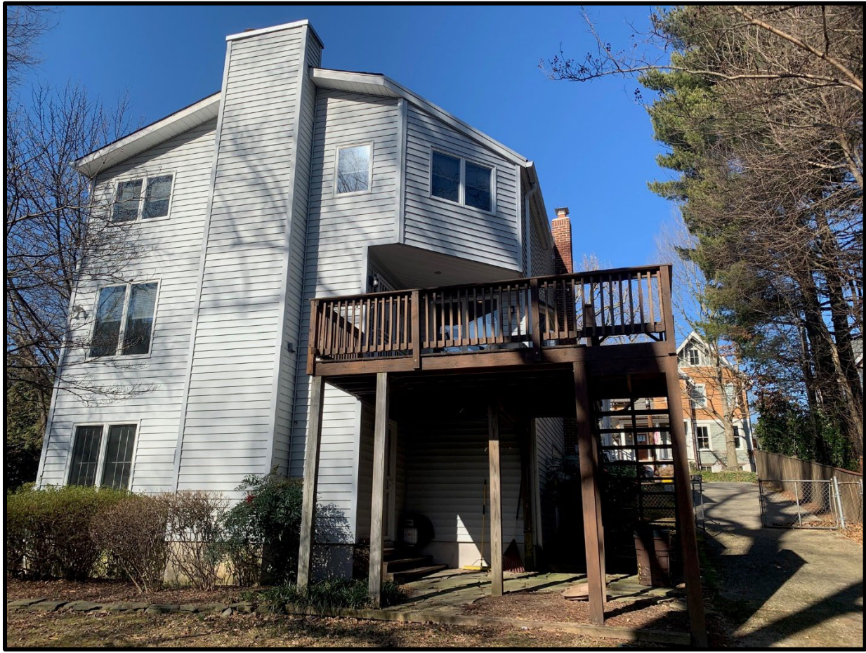
Figure 2: The existing deck and stairs at the rear of 7305 Baltimore Ave.
