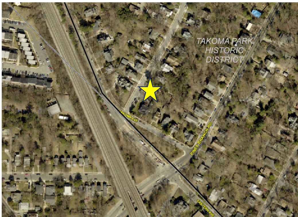
Figure 1: The subject property at 7305 Baltimore Ave. is starred in the Takoma Park Historic District. The district boundaries are outlined in black.
