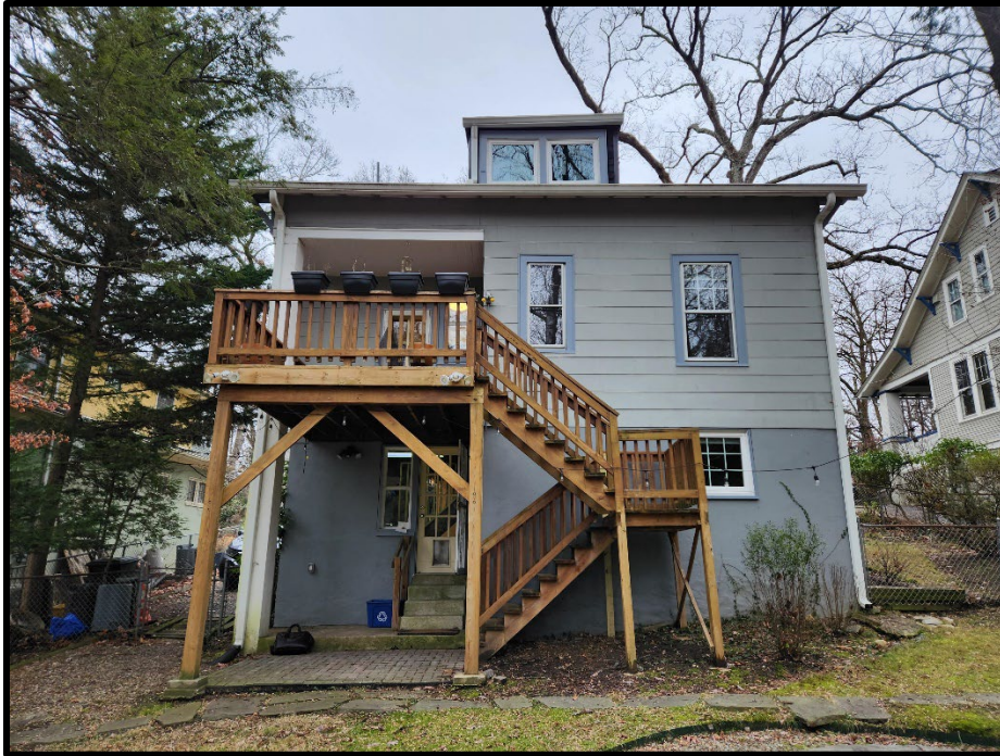
Figure 4: The rear elevation of the subject property. The existing deck is to be removed and replaced with a new deck.
