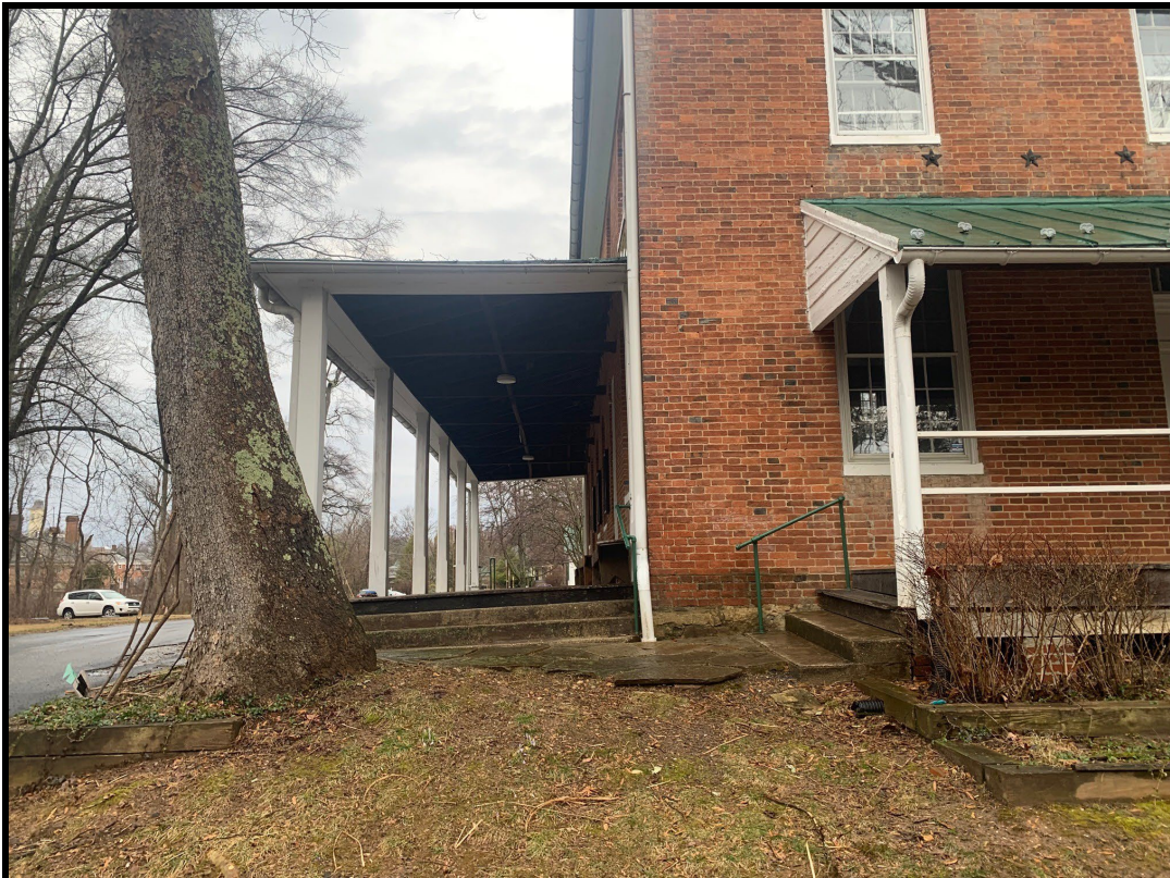
Figure 7. The deck will be installed at this location to link the front porch, left, and the south porch.
