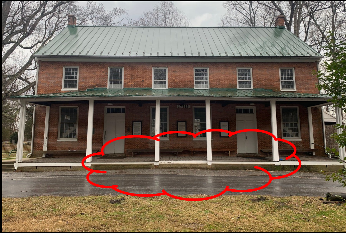
Figure 2. The concrete steps and stair proposed for replacement are clouded in red.
