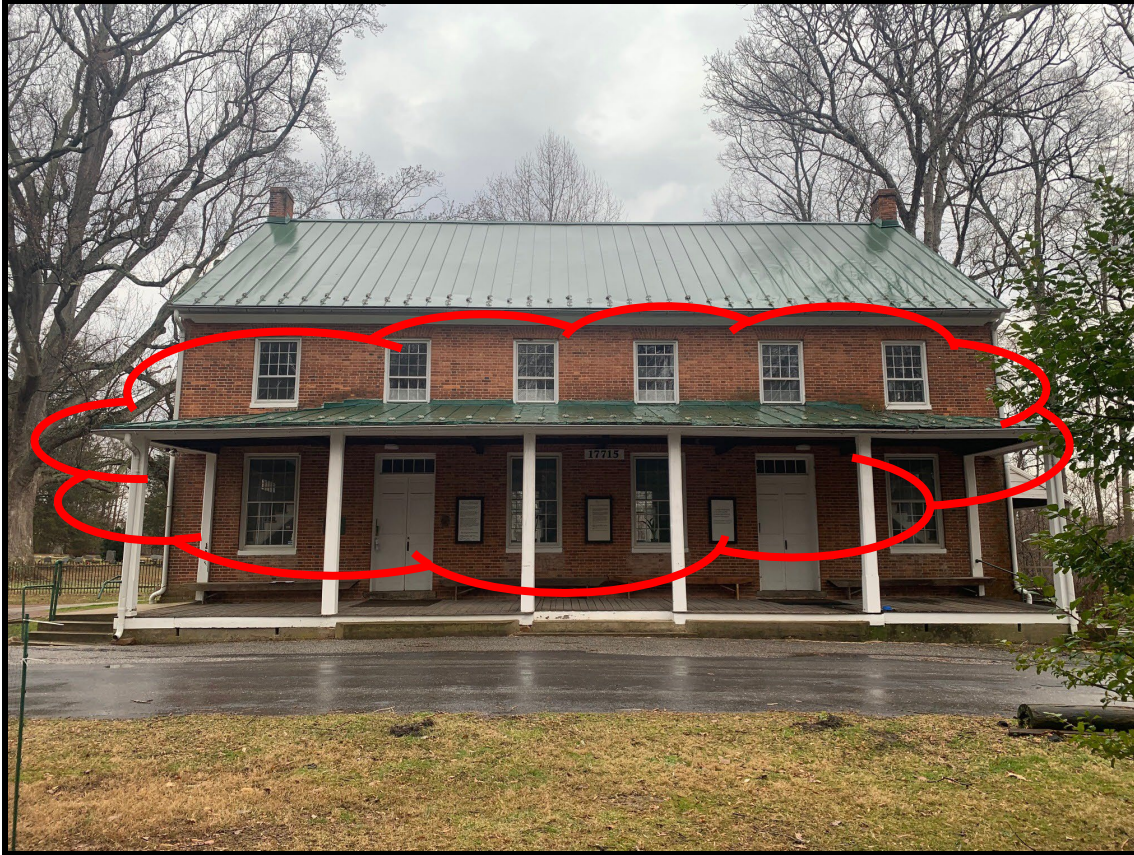
Figure 5. The porch roof proposed for replacement is clouded in red.
