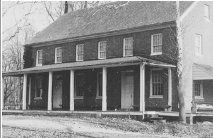
Historic undated photos (Alamy Stock Photos, top. Sandy Spring Digital Archive, bottom.) showing a deck joining the front and south porches. The size of the trees in these photos relative to their size today, dates these photos more than a few decades in the past.
